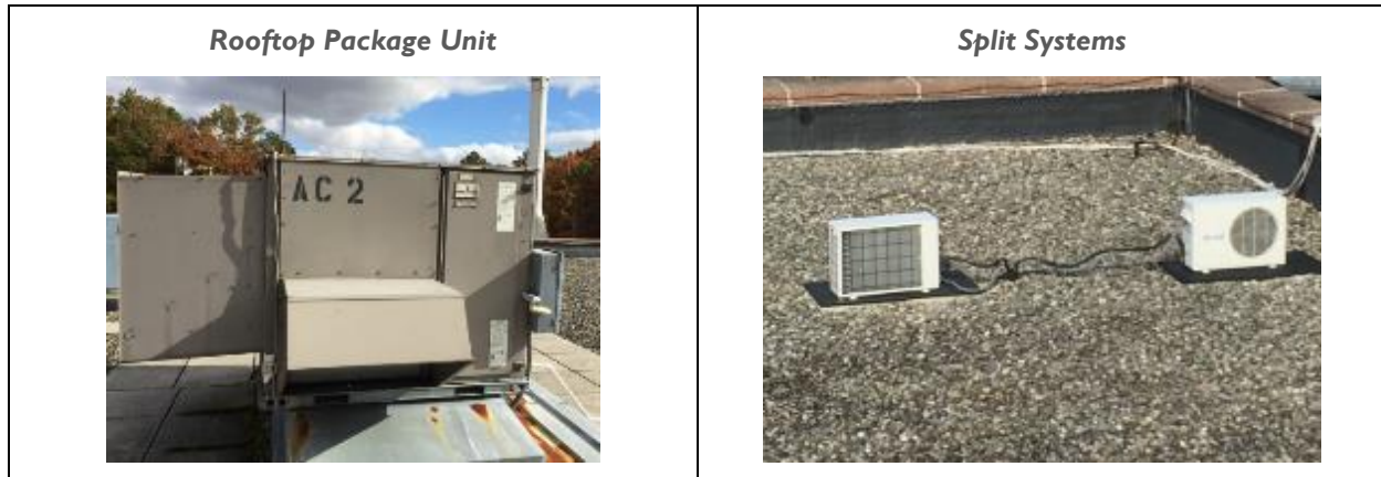
Figure 11 – Direct Expansion AC System
