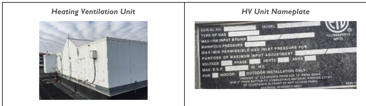
Figure 9 – Air Side Heating System
