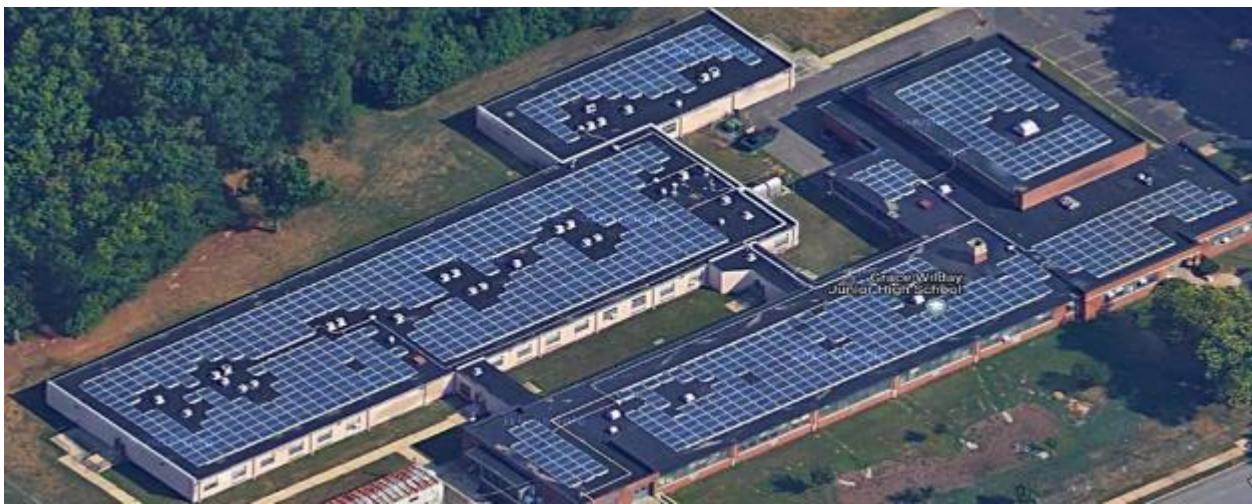
Image 5: Solar PV Arrays
