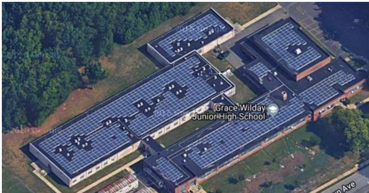
Image 1: Facility Aerial View
