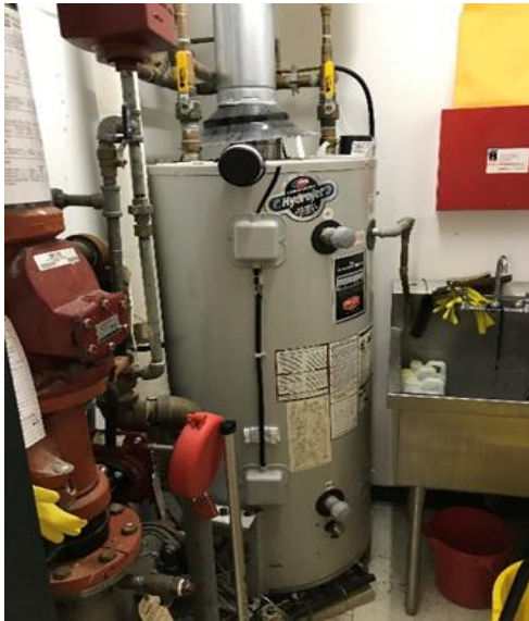
Image 5: Domestic Hot Water Heater
