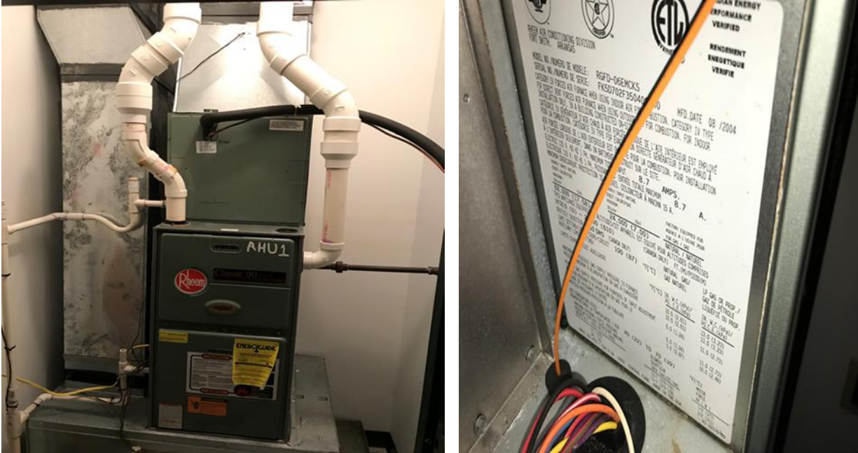
Image 4: Rheem Gas Fired Furnace
