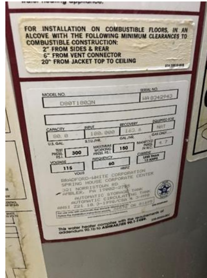
Image 6: Domestic Hot Water Heater nameplate
