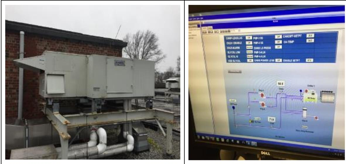
Image 6: AAON RTU & Metasys Chilled Water Control System
