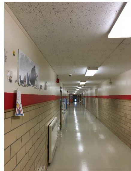
Typical Hallway Lighting
