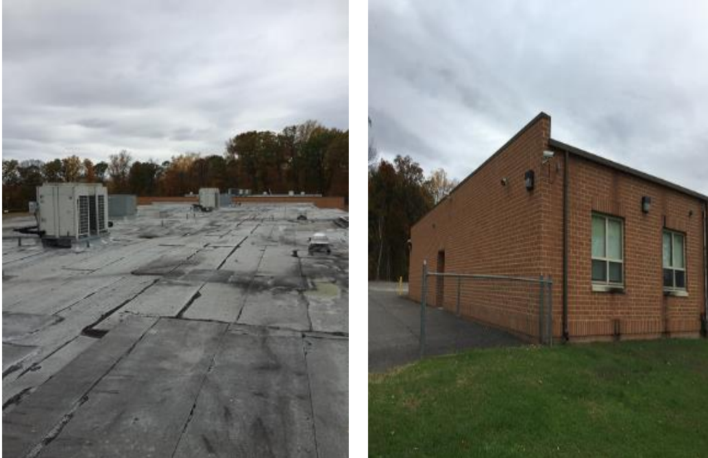
Image 1: Building Wall & Roof
