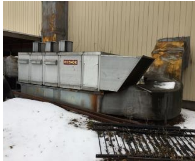
Image 4: Reznor Gas Fired Furnace
