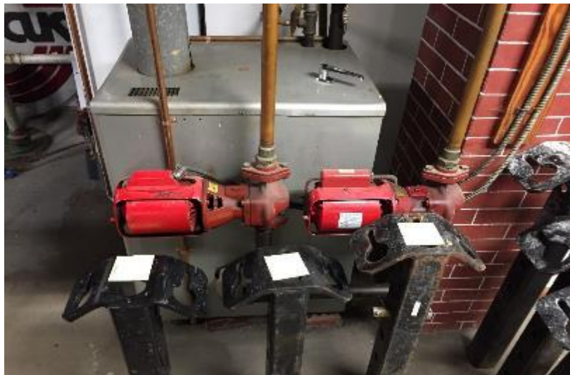
Figure 7: Hot Water Boiler
