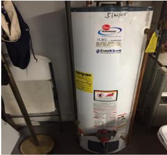
Image 5: Gas Fired Water Heater
