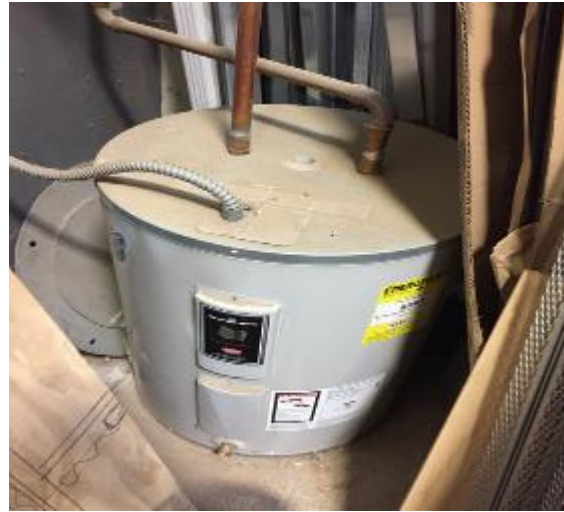
Image 6: Electric Water Heater
