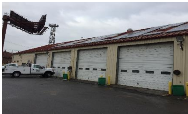
Image 2: DPW Garage Building
