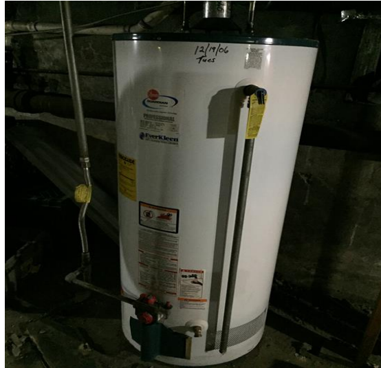
Image 3: Domestic Hot Water
