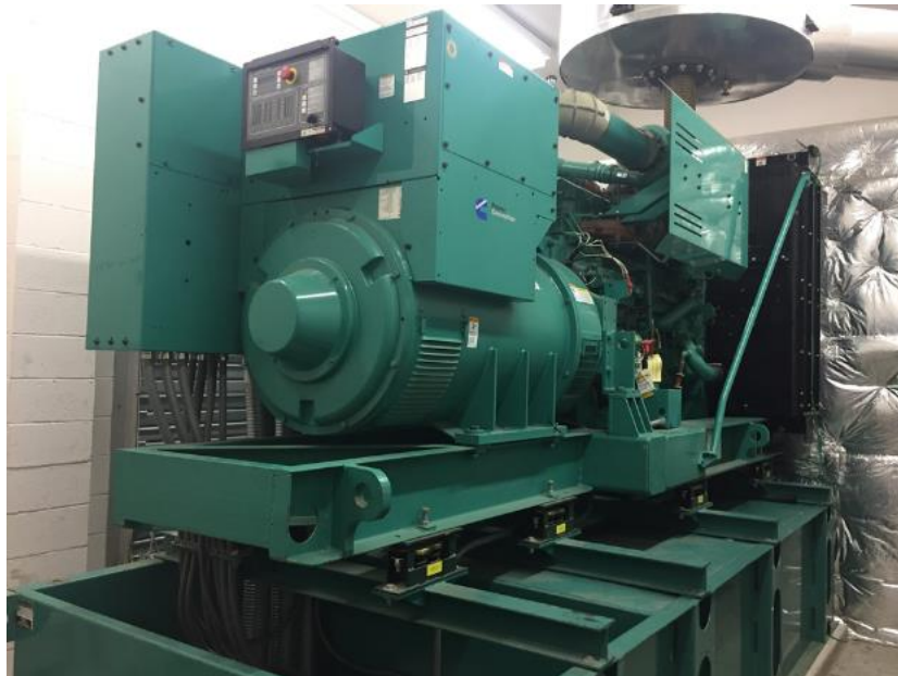
Image 4: Cummins Diesel Engine Generator
