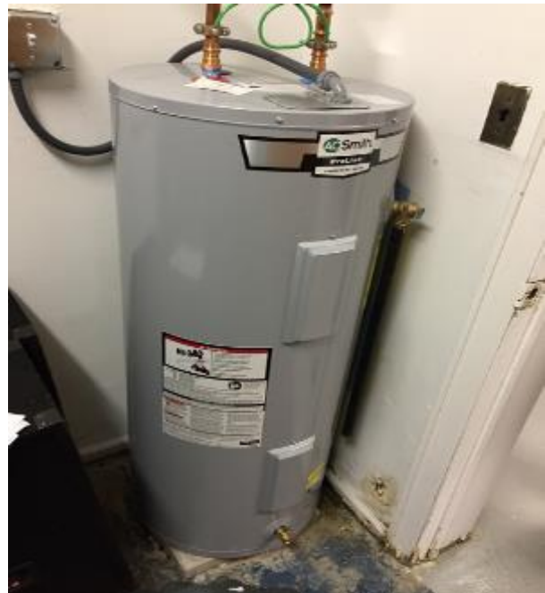
Image 9: Electric Water Heater
