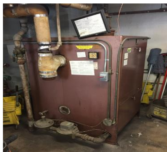
Image 3: Old & Inefficient Hot Water Boiler
