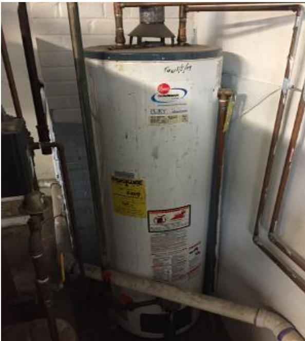
Image 8: Gas Fired Water Heater
