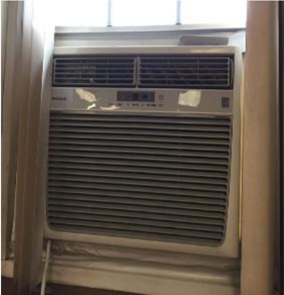
Image 5: Typical Window Unit
