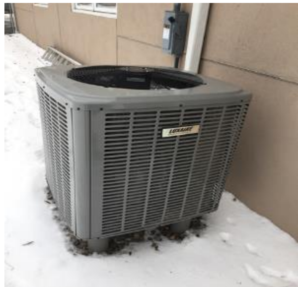
Image 3: Split AC Condensing Unit
