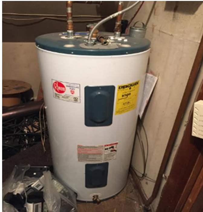
Image: Domestic Water Heater
