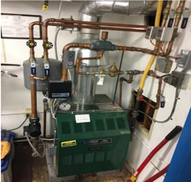
Image 2: Genesis Hot Water Boiler
