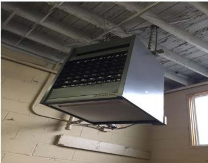
Image 4: Sterling Gas Fired Unit Heater
