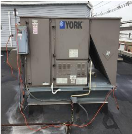
Image 5: York Packaged AC & Programmable Thermostats
