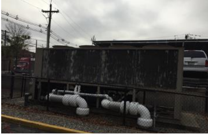
Image 4: York Air-Cooled Chiller
