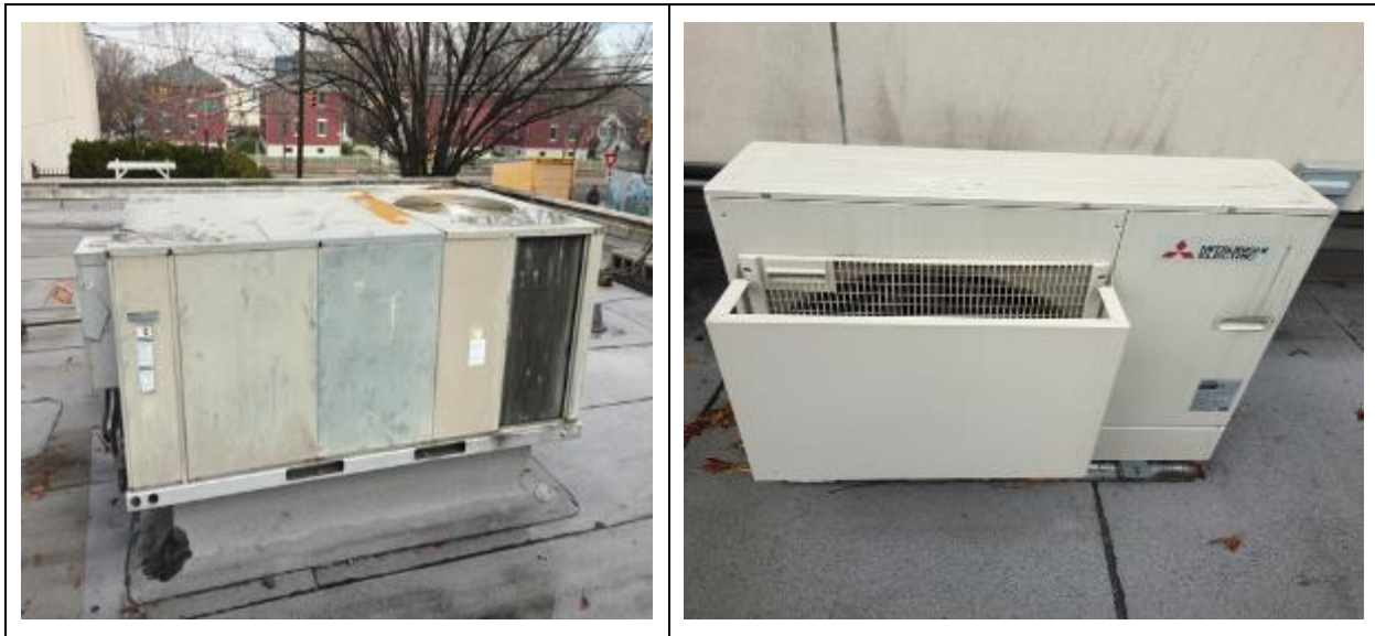
Image 6: Direct Expansion System
