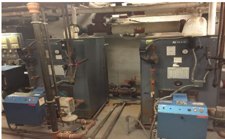
Image 3: Hot Water Boilers
