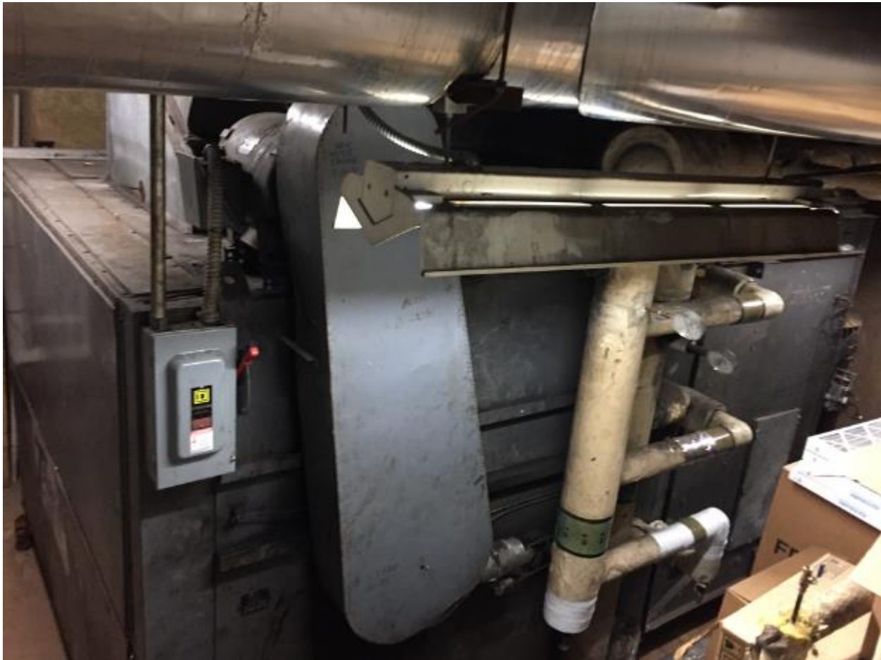
Image 5: Old Air Handler Unit
