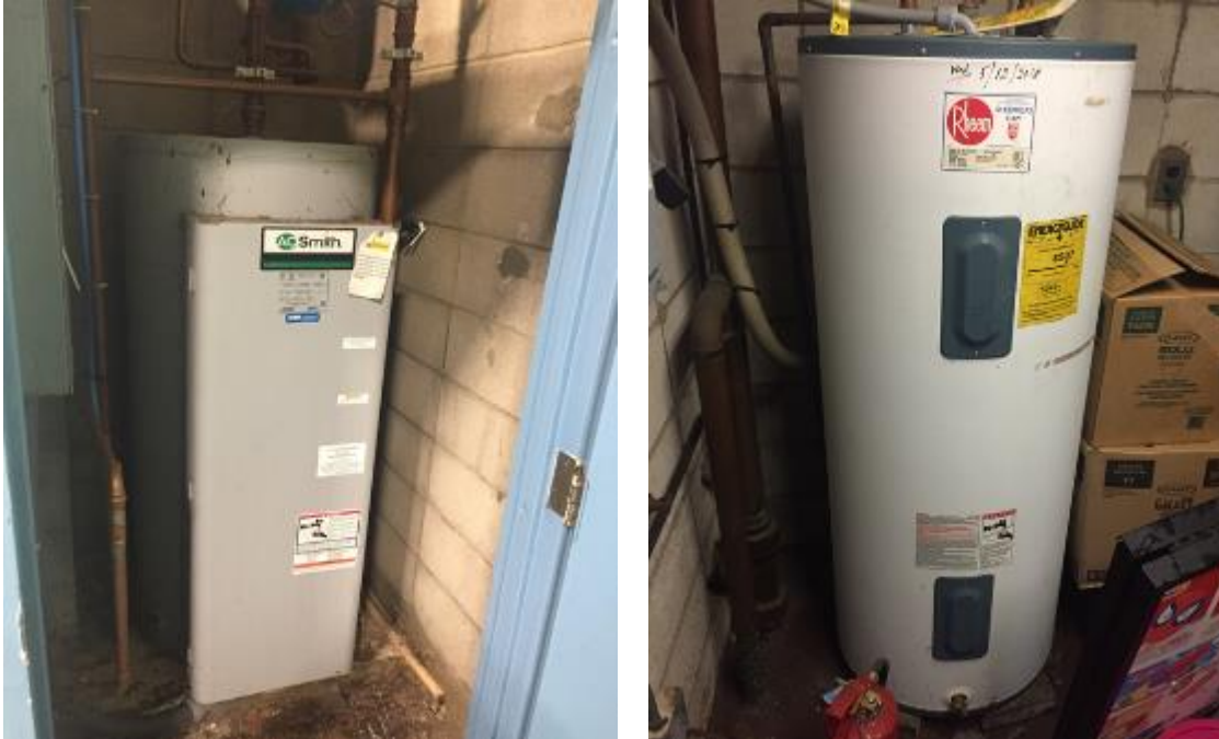
Image 4: Domestic Water Heaters
