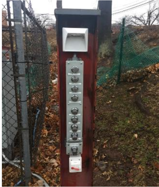
Image 2: Lighting Control Manual Switches
