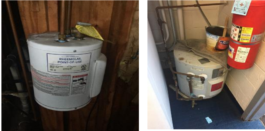
Image 3: Domestic Water Heaters
