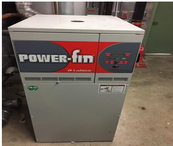
Image 7: Domestic Hot Water Heater
