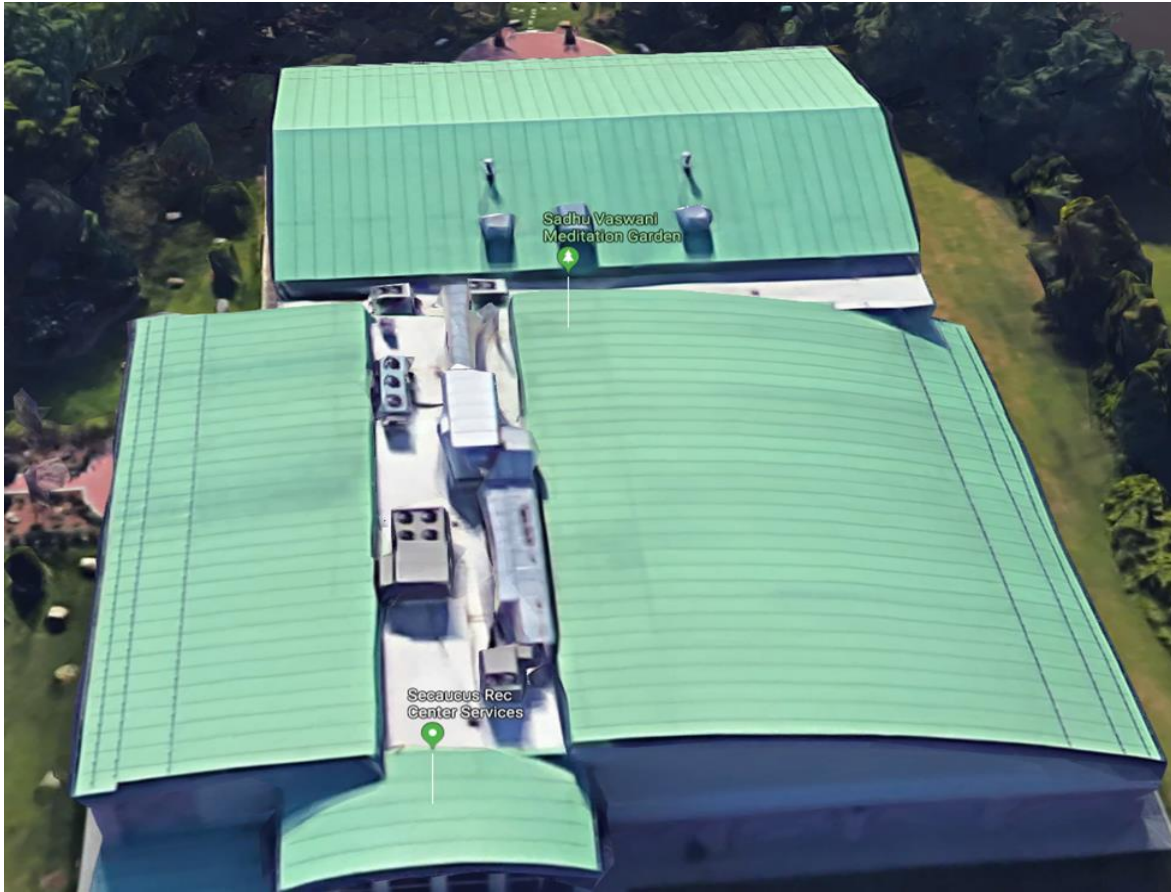
Image 9: Aerial View of the Free Rooftop Spaces
