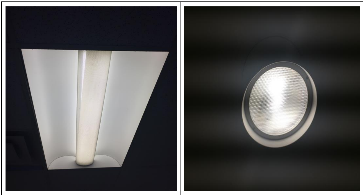
Image 3: Interior Lighting System
