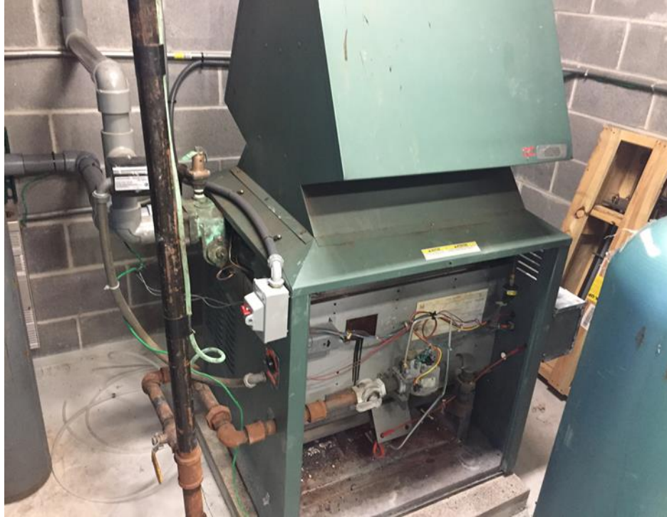
Image 4: Indoor Pool Hot Water Boiler
