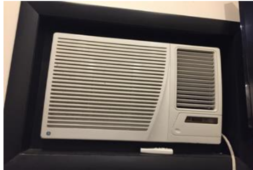
Image 1: Typical Window AC
