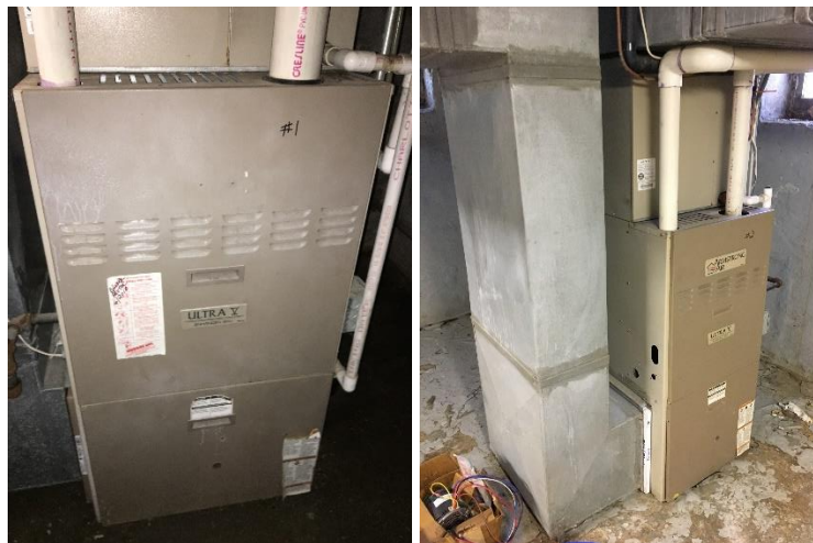
Image 4 Heat and AC systems at the Admin Building
