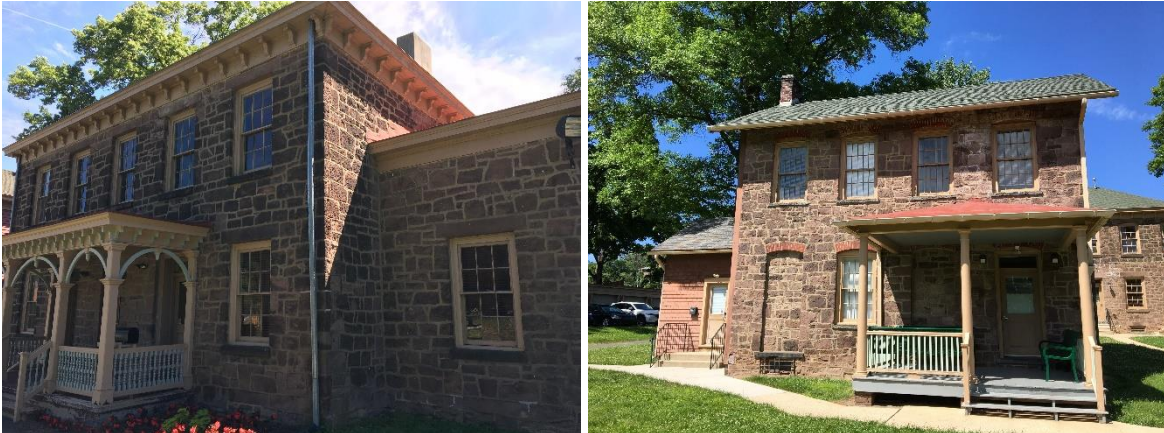
Image 1 Left: Admin Building Envelope, Right: Cottage Art Barn
