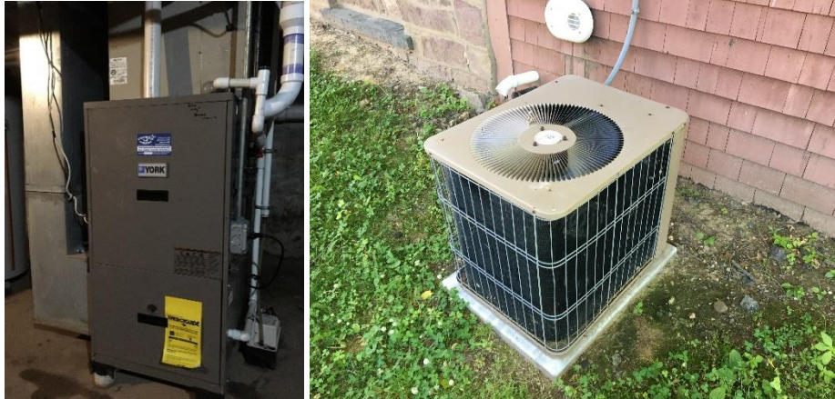
Image 5 Heat and AC system at the Cottage Art Barn
