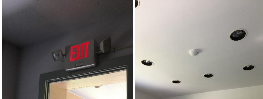
Image 3 Lighting System at the Cottage Art Barn
