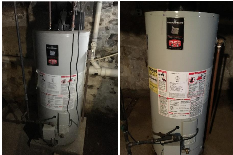
Image 6 Domestic Hot Water Systems
