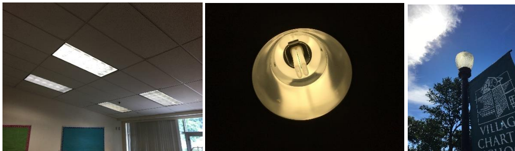
Image 2 Typical Lighting Fixtures
