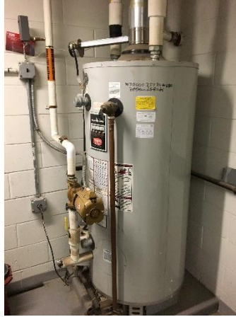
Image 5 Domestic Hot Water Heating System
