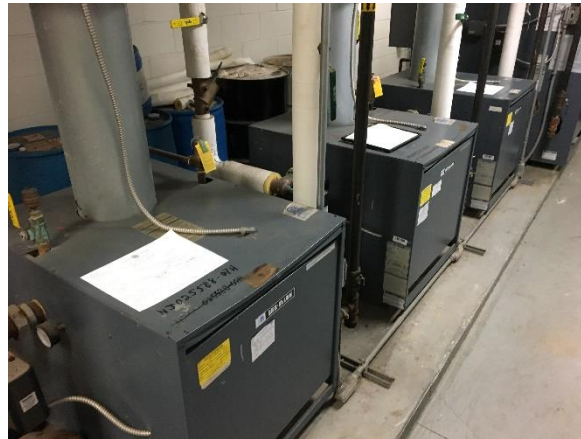
Image 3 Hot water heating system
