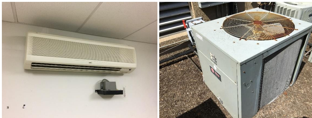
Image 4 DX cooling system
