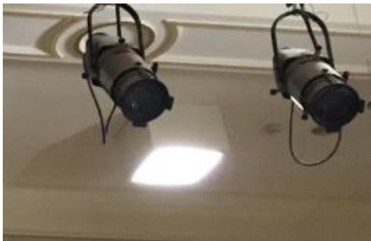
Auditorium LED and Halogen Incandescent Lamps
