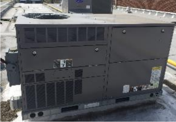
4-ton Packaged AC Unit
