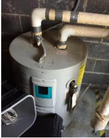
State 40-gal Electric DHW Heater
