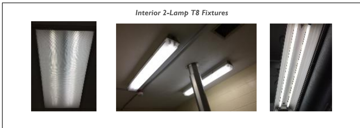
Figure 8 - Building Lighting Systems
