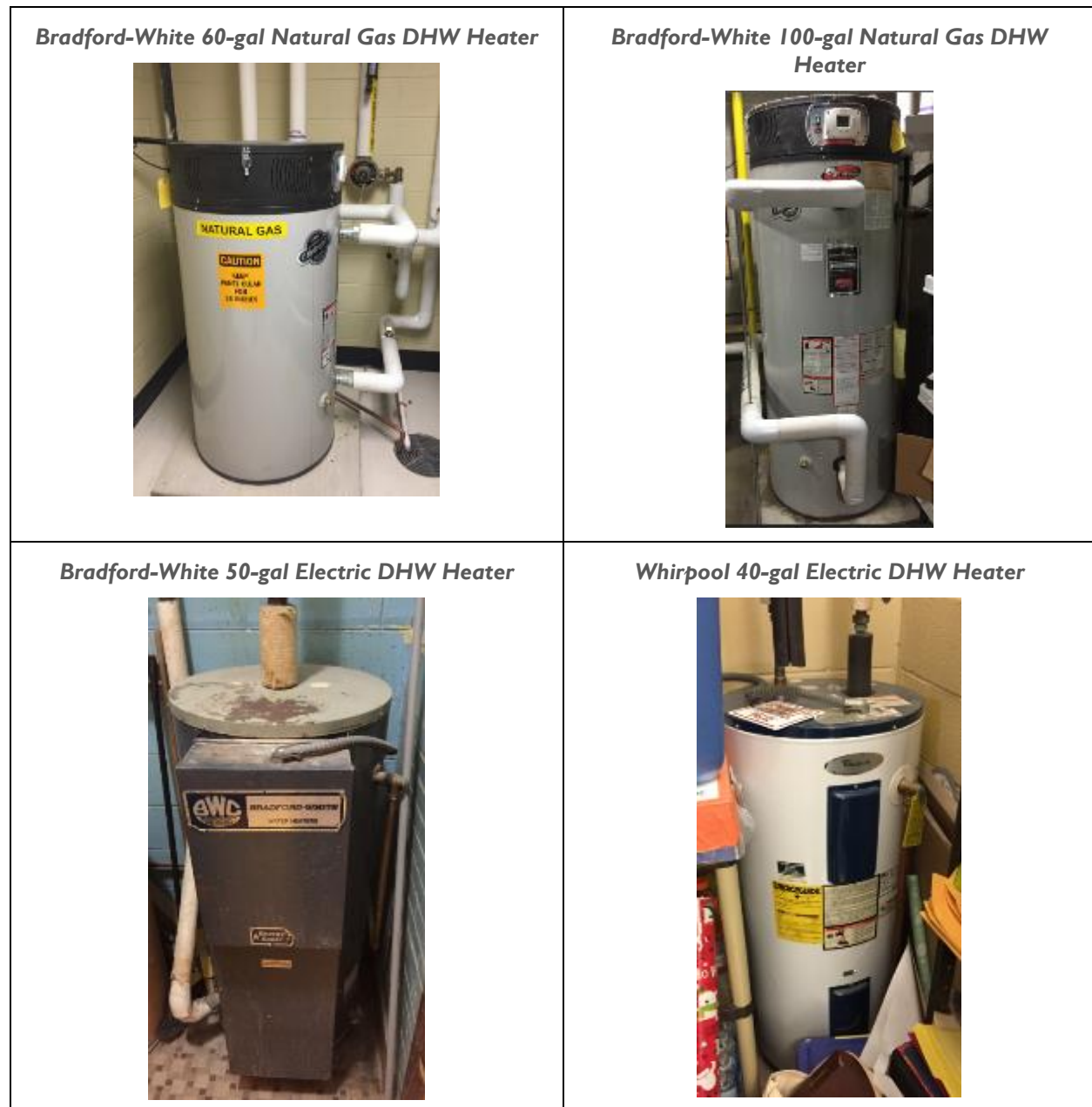
Figure 11 - Domestic Hot Water System
