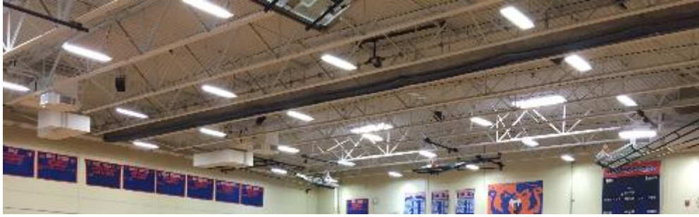
Interior 4-Lamp T5 Fixtures
