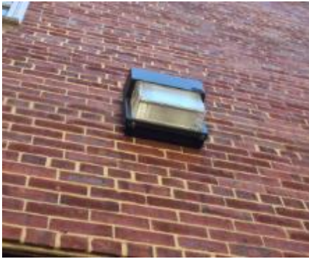
Exterior MH Wall-Mounted Fixture
