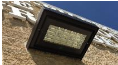
Exterior LED Fixtures
