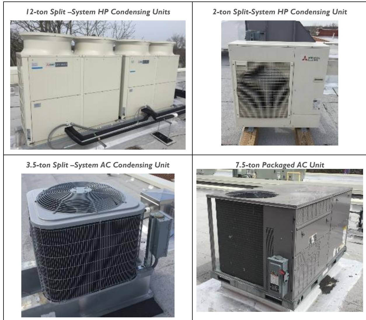
Figure 10 - Building AC Systems
