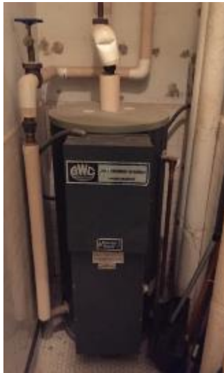
Bradford-White 50-gal Electric DHW Heater
