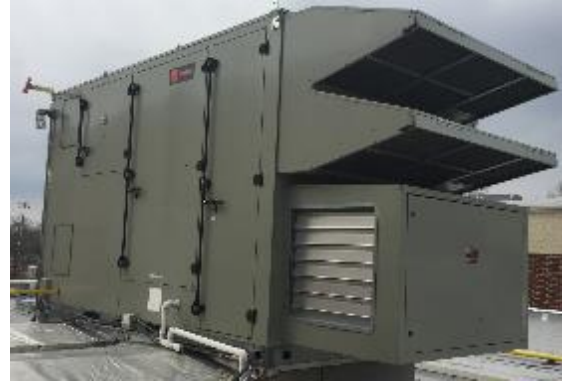
54-ton Packaged AC Unit
