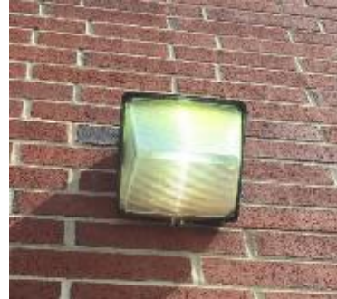
Exterior HPS Fixture
