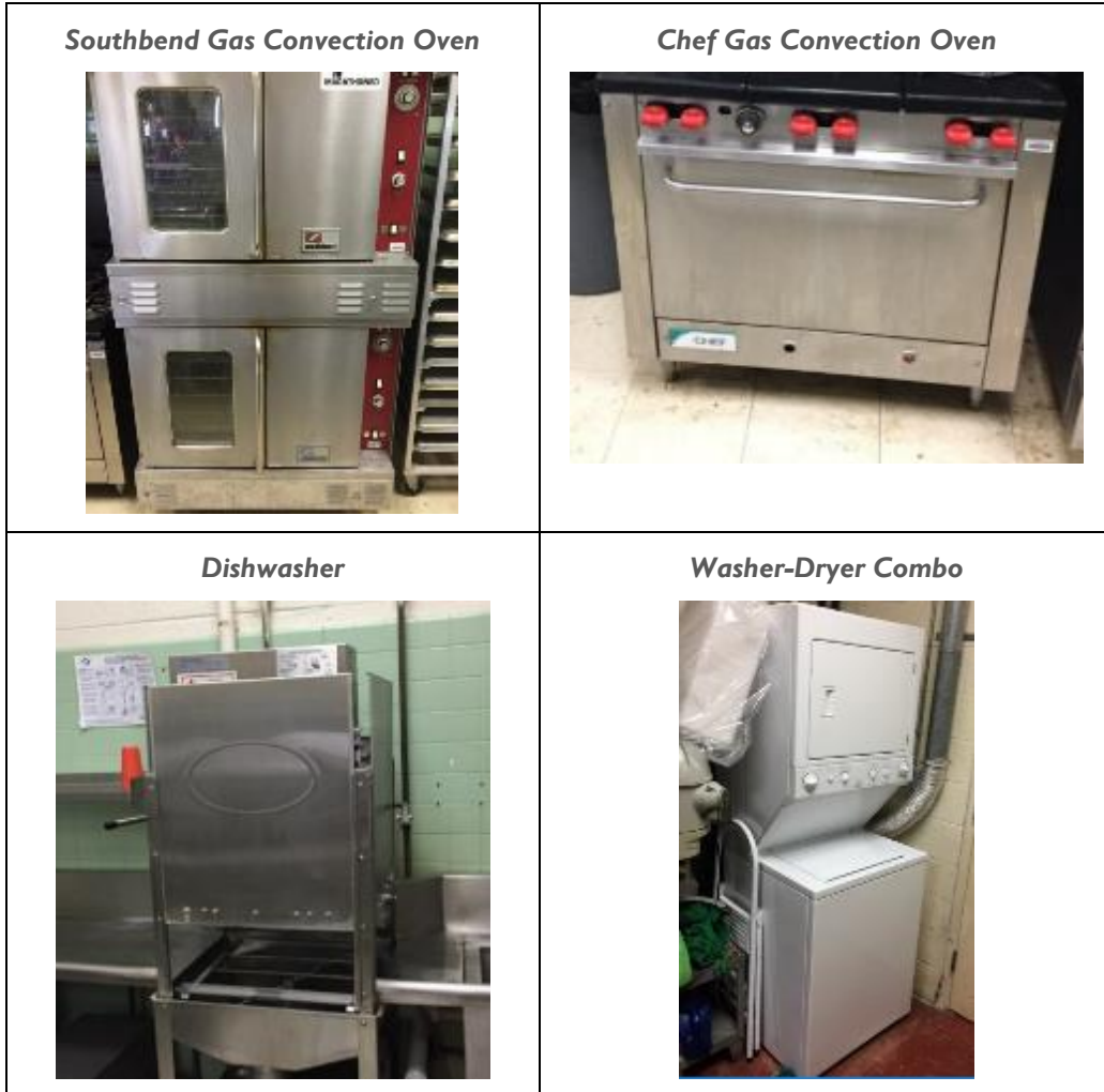
Figure 12 – Food Service and Laundry Equipment
