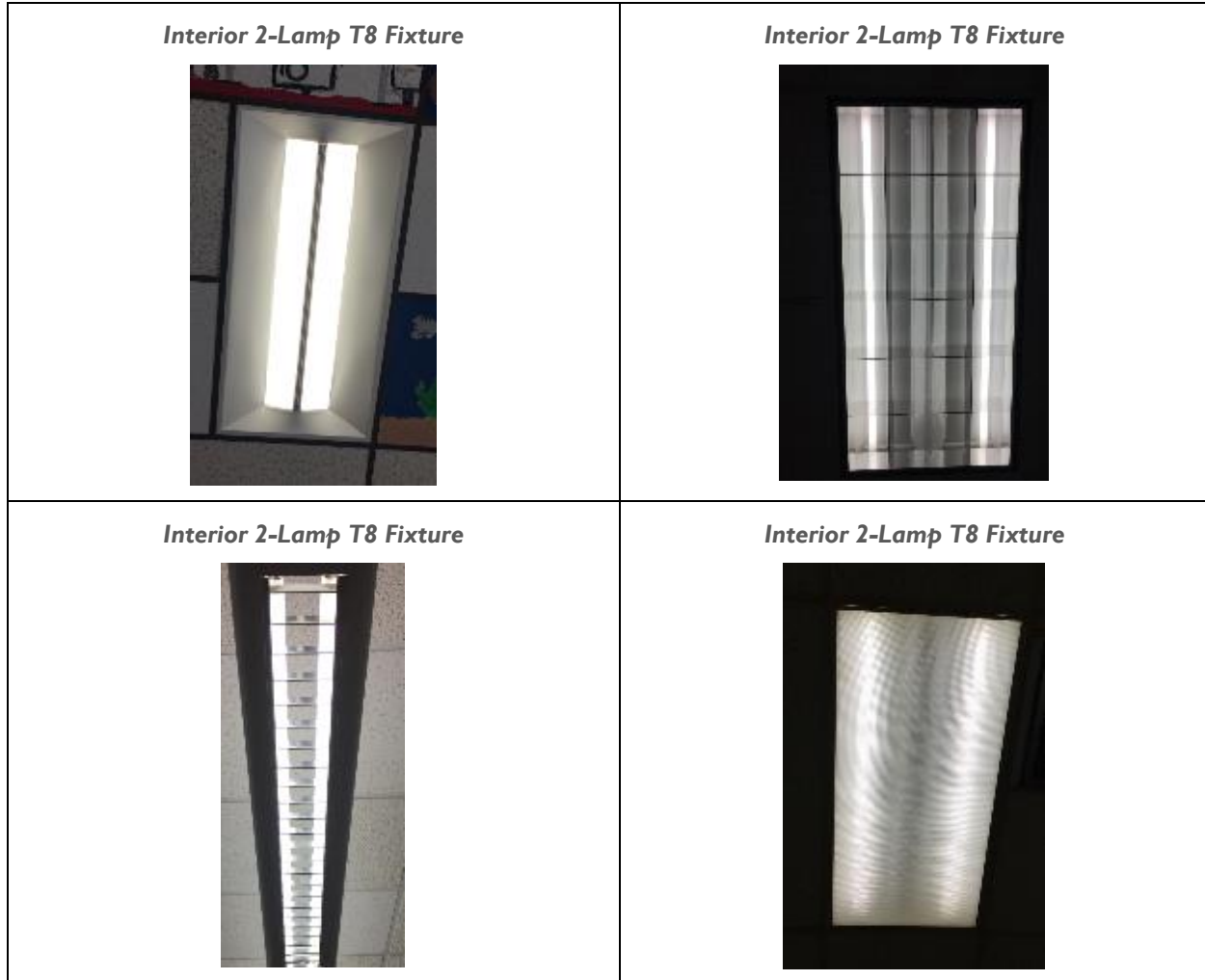
Figure 8 - Building Lighting Systems
