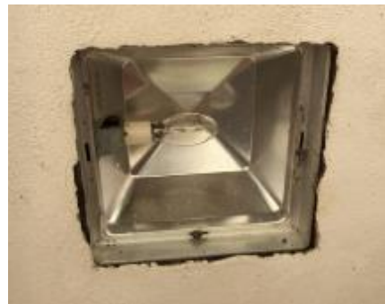
Exterior HPS Fixture
