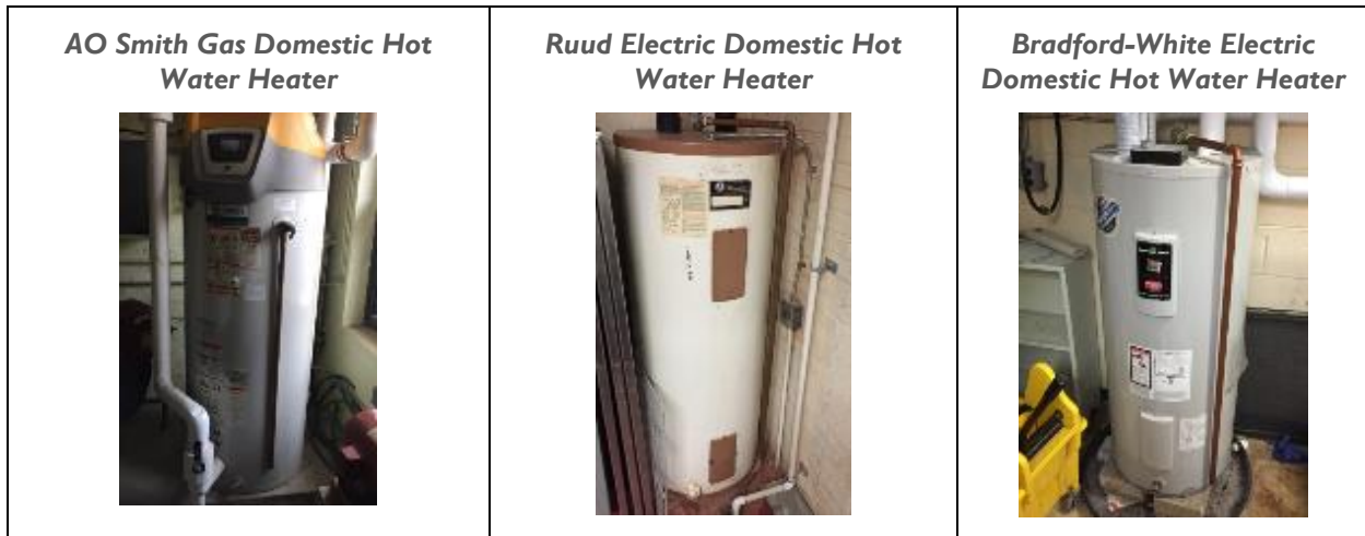
Figure 11 - Domestic Hot Water System
