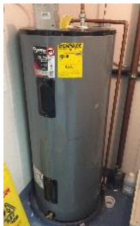
Figure 10 - Domestic Hot Water Heater
