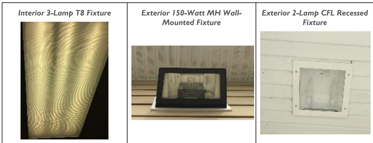
Figure 8 - Building Lighting Systems
