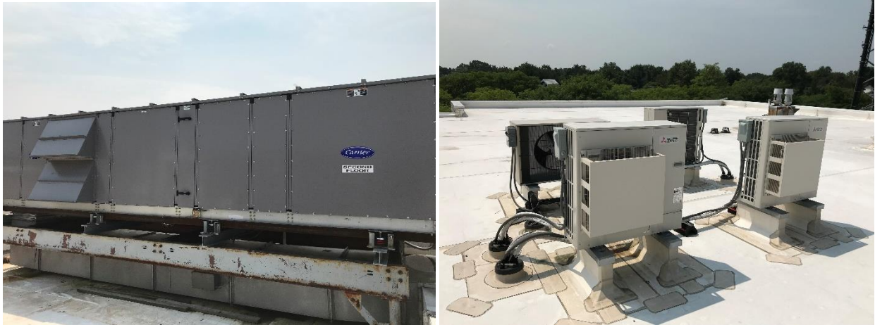
Image 5 AHU & DX Systems on Roof
