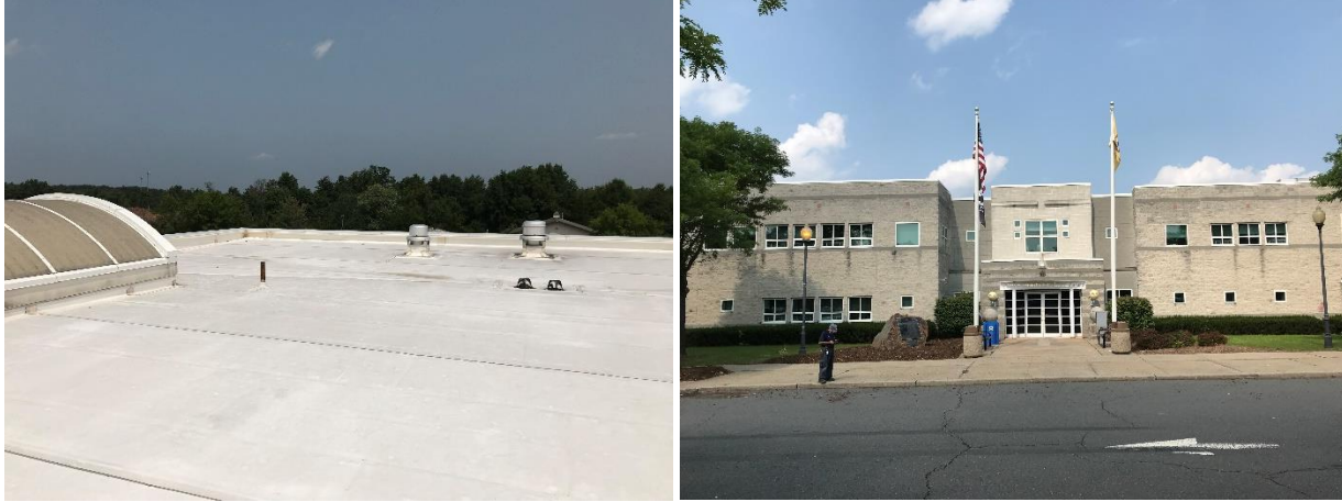
Image 1 Building Roof and Exterior
