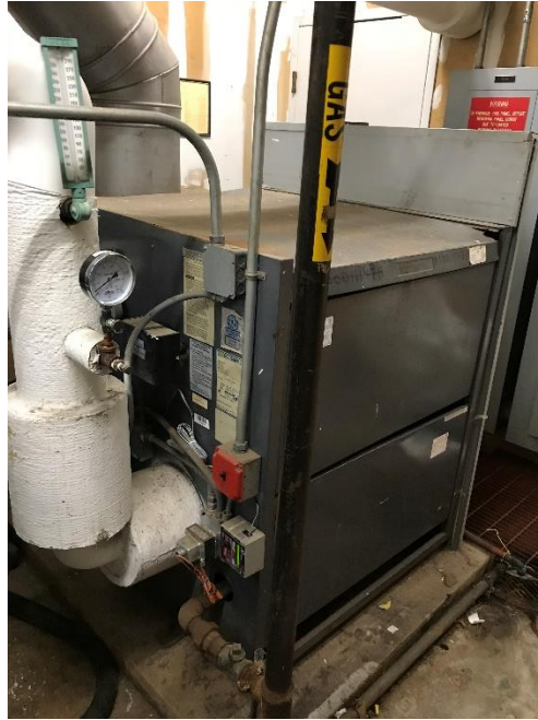
Image 4 Hot Water Boiler system
