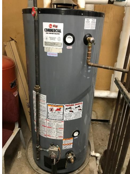
Image 7 DHW Heater with Storage Tank
