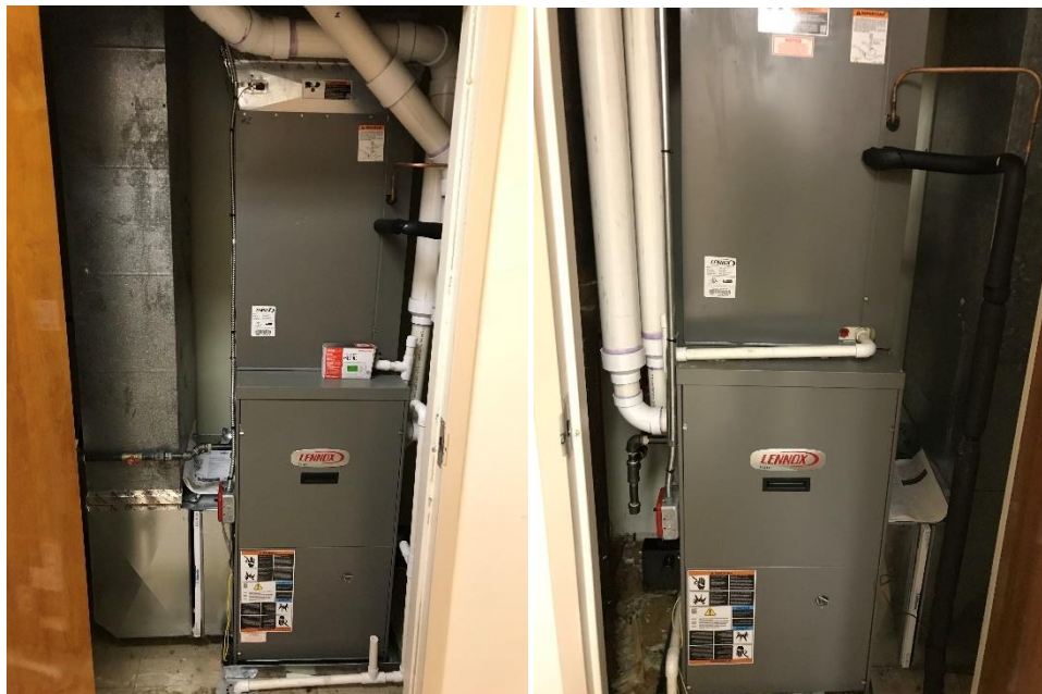
Image 3 Indoor Gas fired furnaces
