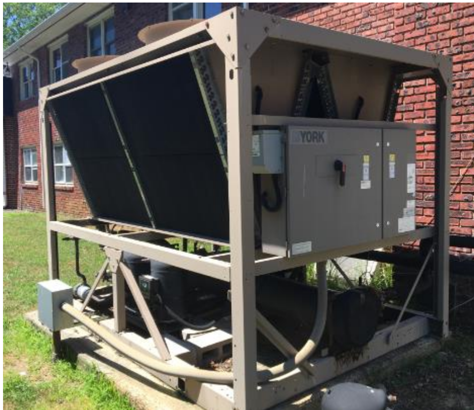
Image 13. York Air Cooled Chiller
