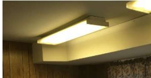
Image 4. Ceiling Mount Linear Fluorescent Fixture
