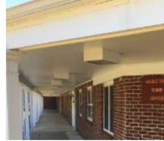
Image 9. Ceiling Mounted Canopy Fixtures
