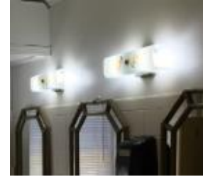
Image 5. Wall Mount Lighting in Restroom
