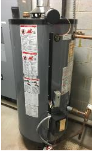
Image 14. Picture of the 75- Gallon Water Heater
