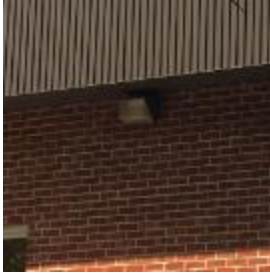
Image 7. Exterior Wallpack Fixture
