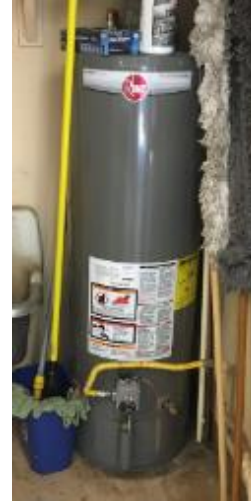
Image 15. Picture of the 40-Gallon Water Heater
