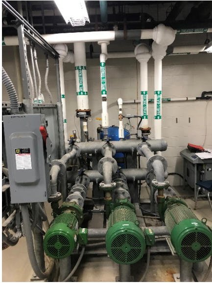
Image 17 Hot water circulation Pumps
