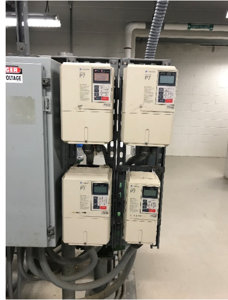
Image 18 VFDs for HW pumps
