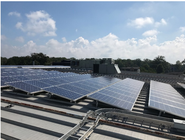
Image 29 Solar Plant on roof
