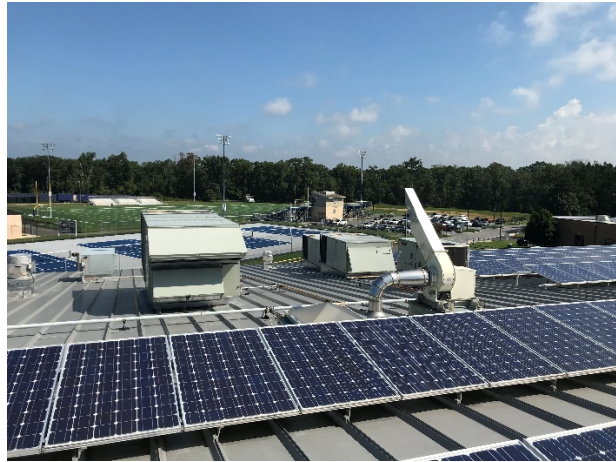
Image 12 RTUs on roof
