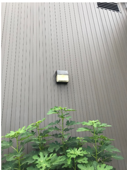
Image 9 Outdoor wall mounted fixtures
