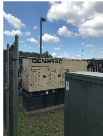
Image 30 Outdoor Emergency Generator
