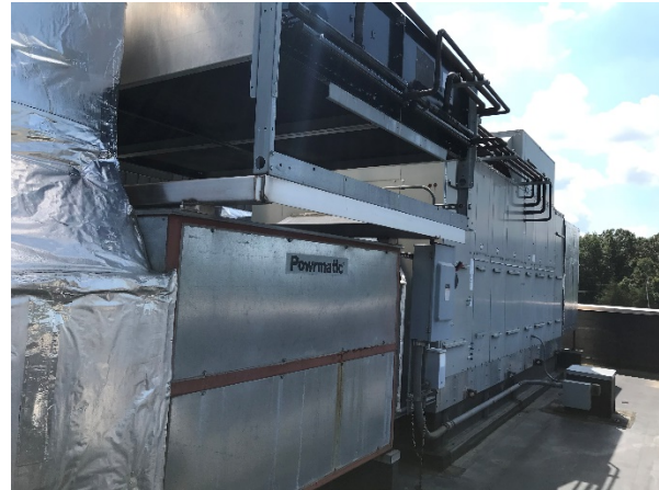
Image 14 Poolpack dehumidifier
