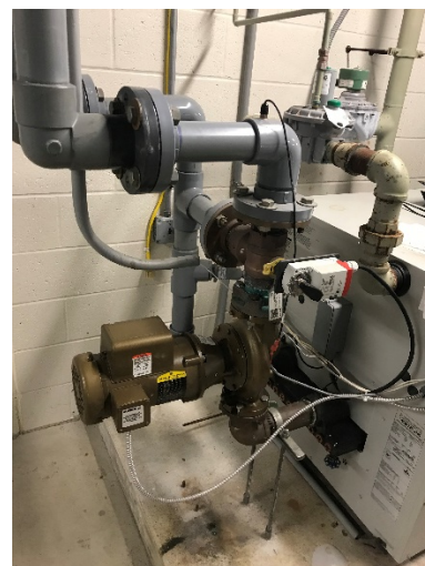
Image 16 Water supply pump
