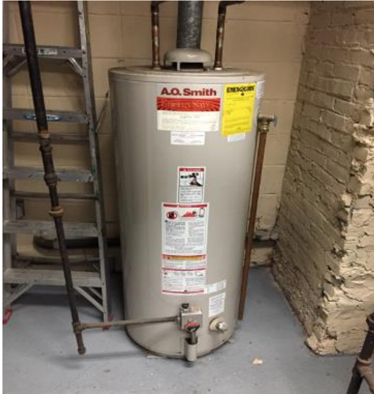
Image 6: Domestic Water Heater
