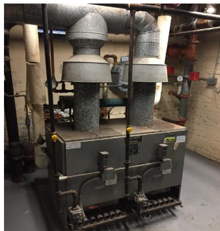
Image 3: Hot Water Boiler
