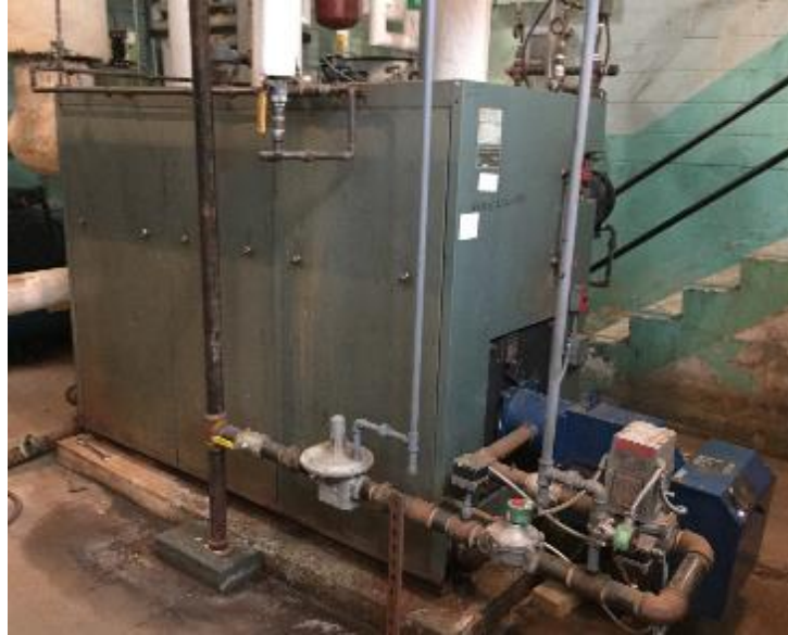
Figure 11 - Picture of the steam boiler
