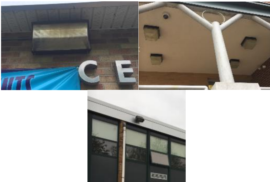
Figure 9 - Pictures of the various exterior HID lighting
