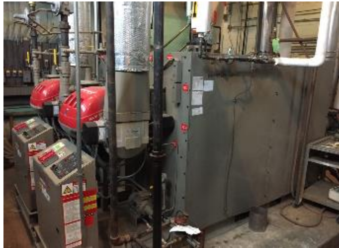
Figure 10 - Picture of the condensing boilers
