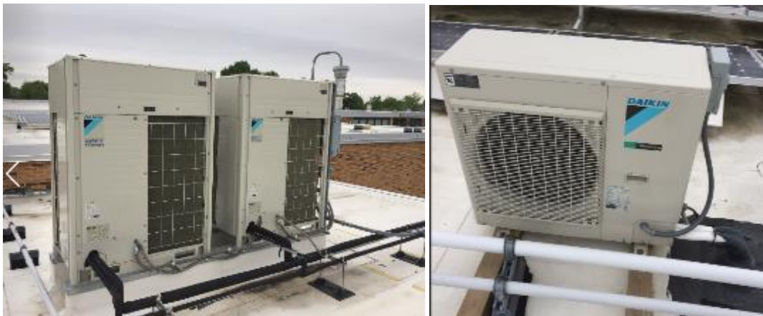
Figure 12 - Pictures of some of the condensing units of heat pumps and air conditioning units
