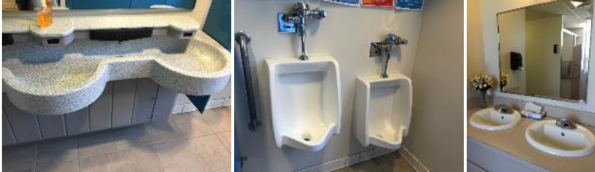
Image 5 Water using systems at the facility
