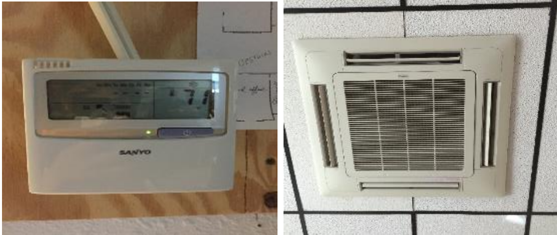
Image 4 Typical air-conditioning equipment found at the site
