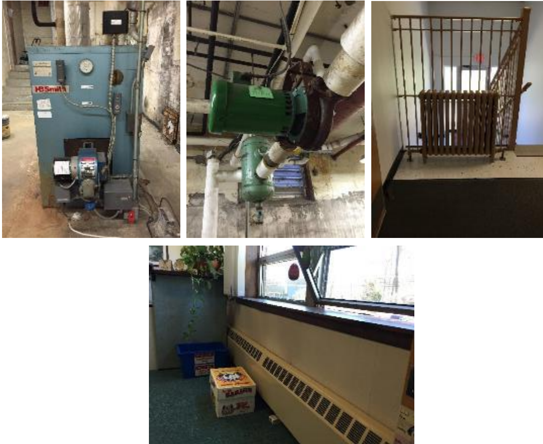
Image 3 Hot water heater and circulating pump
