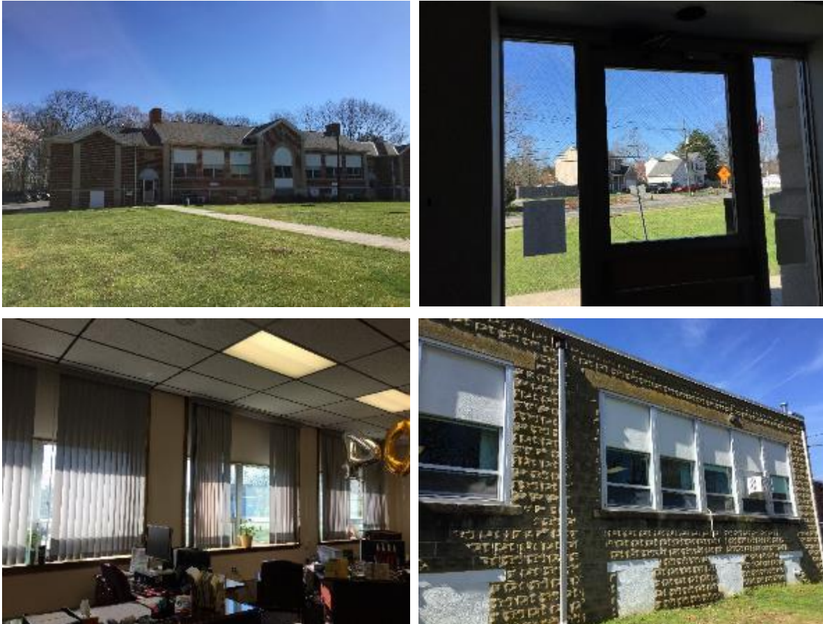
Image 1 Images of the building envelope
