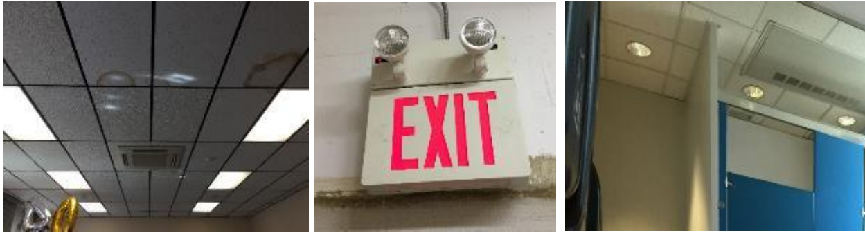
Image 2 Lighting fixtures at the building
