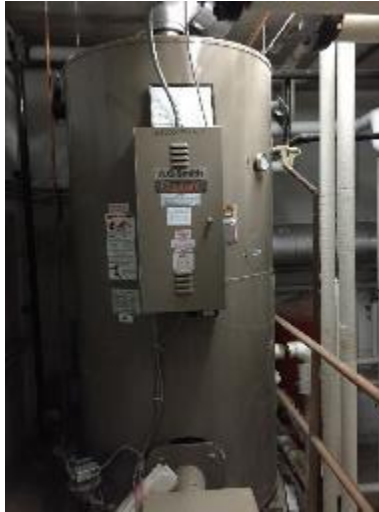
Image 5 – Domestic Hot Water
