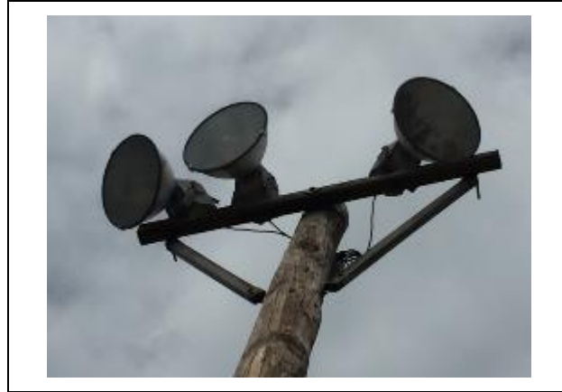
Figure 7 - Meyersville Ballfield Lighting Systems
