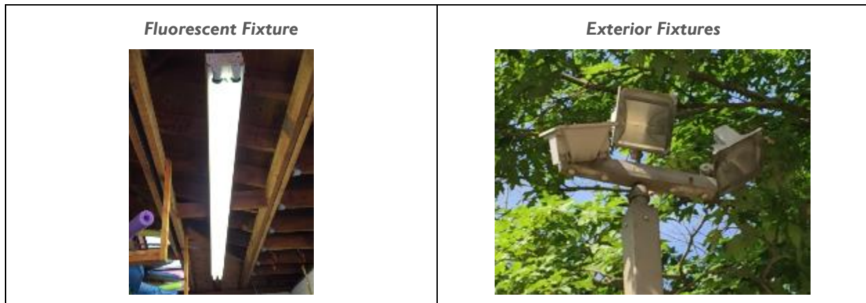
Figure 8 - Stirling Lake Lighting Systems
