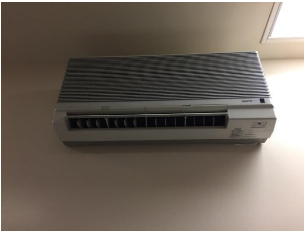
Image 5 Split System indoor (evaporator)
