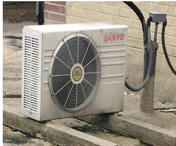
Image 6 Split System outdoor (condenser)
