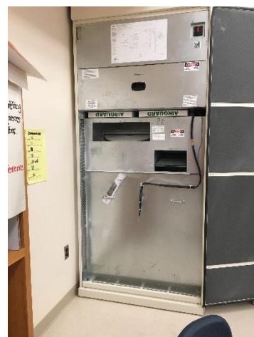
Image 8 In-classroom package unit w/HW coil
