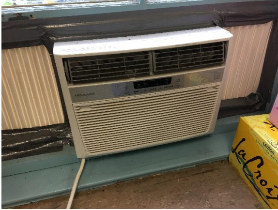
Image 7 – Typical window AC unit
