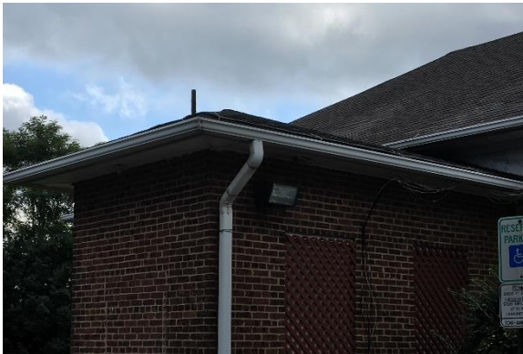
Image 5 – Exterior metal halide wall pack
