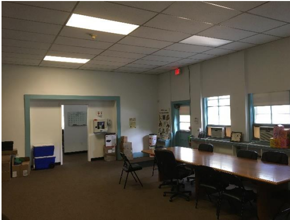
Image 3 – Typical T8 4' & 2' fluorescent fixtures
