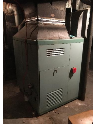
Image 8 – Oil fired furnace
