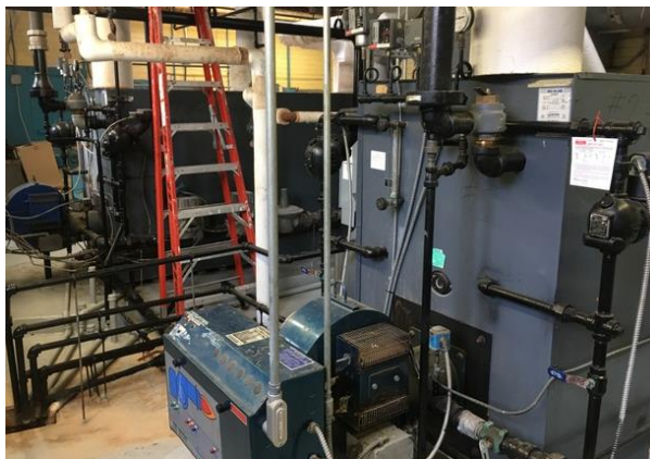
Picture 4: Steam Boilers
