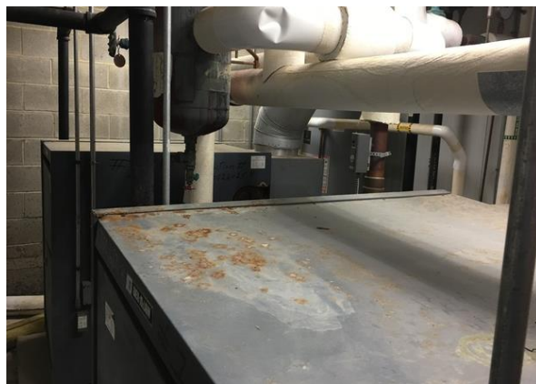
Picture 5: Hot Water Boilers
