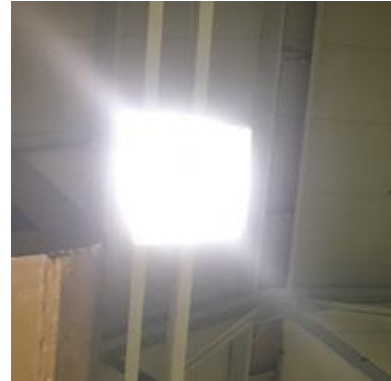
Picture 3: HID Fixture
