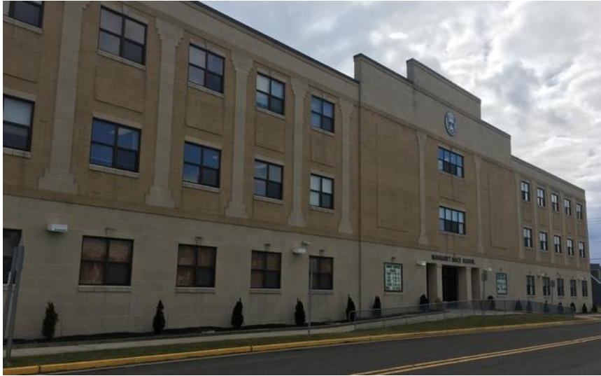
Picture 1: Building Exterior
