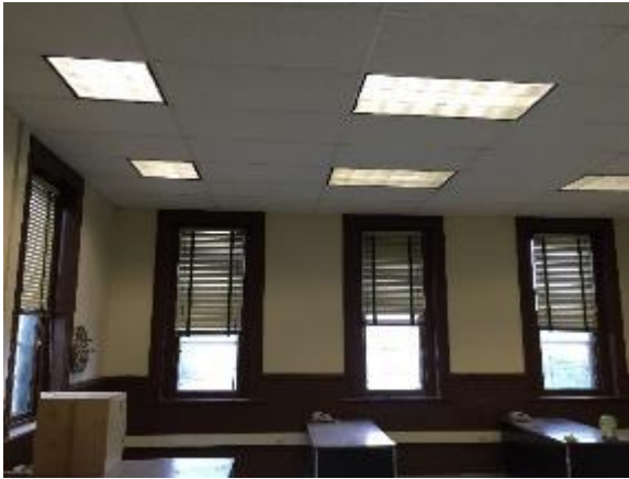
Image 2 – Typical linear fluorescent fixtures
