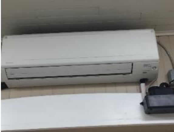
Image 4 – Indoor unit (ductless heat pump fan coil)
