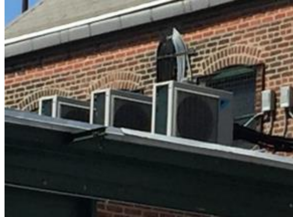
Image 5 – Outdoor units (condensers)
