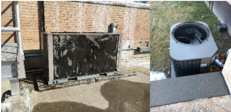
Image 21: Remote Condensing Units
