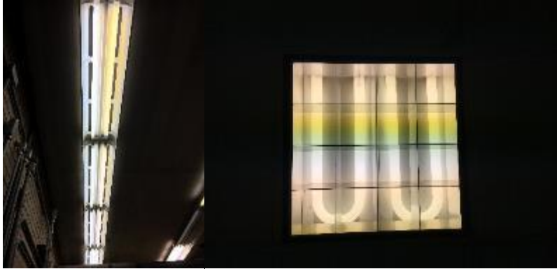
Image 2: Interior Linear Fluorescent T12 Light Fixtures
