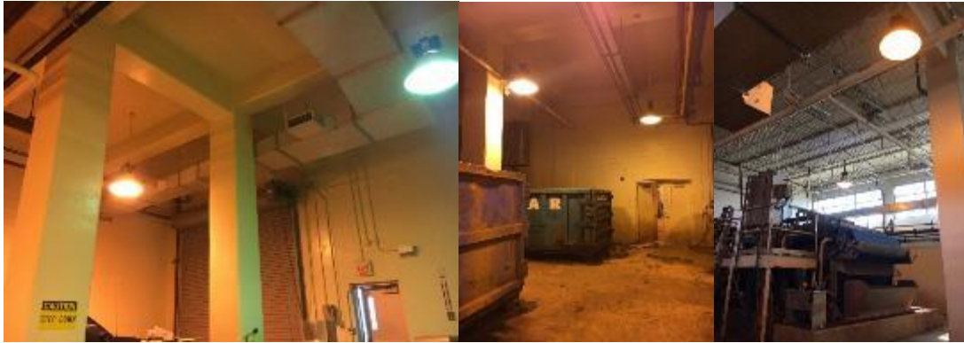
Image 5: High Bay HID Lighting in Mechanical Dewatering Facility
