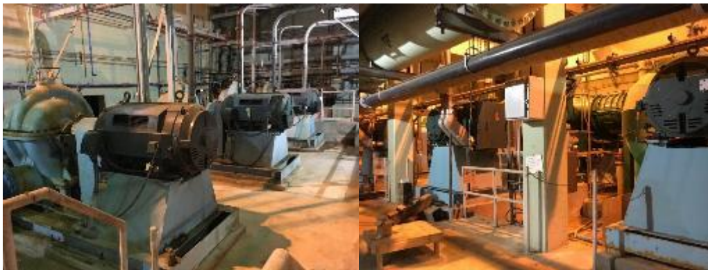
Image 7: Raw Water and High Service Pump Motors
