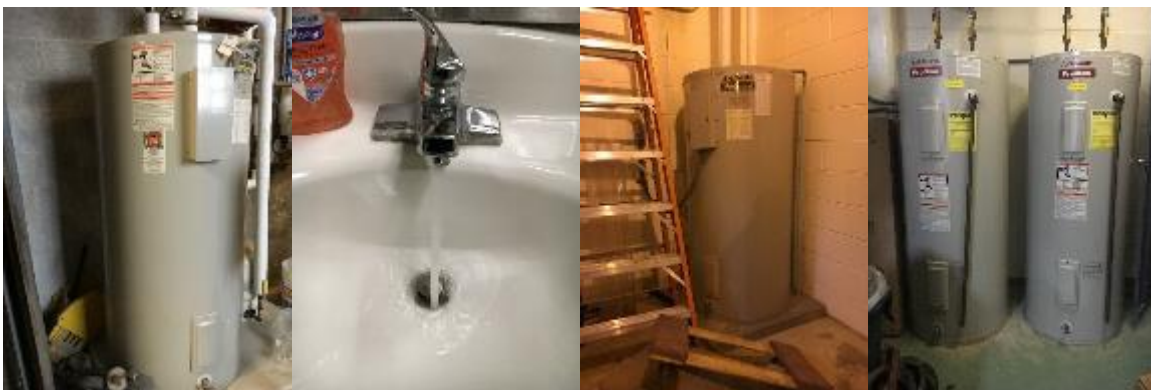
Image 23: Domestic Hot Water Systems
