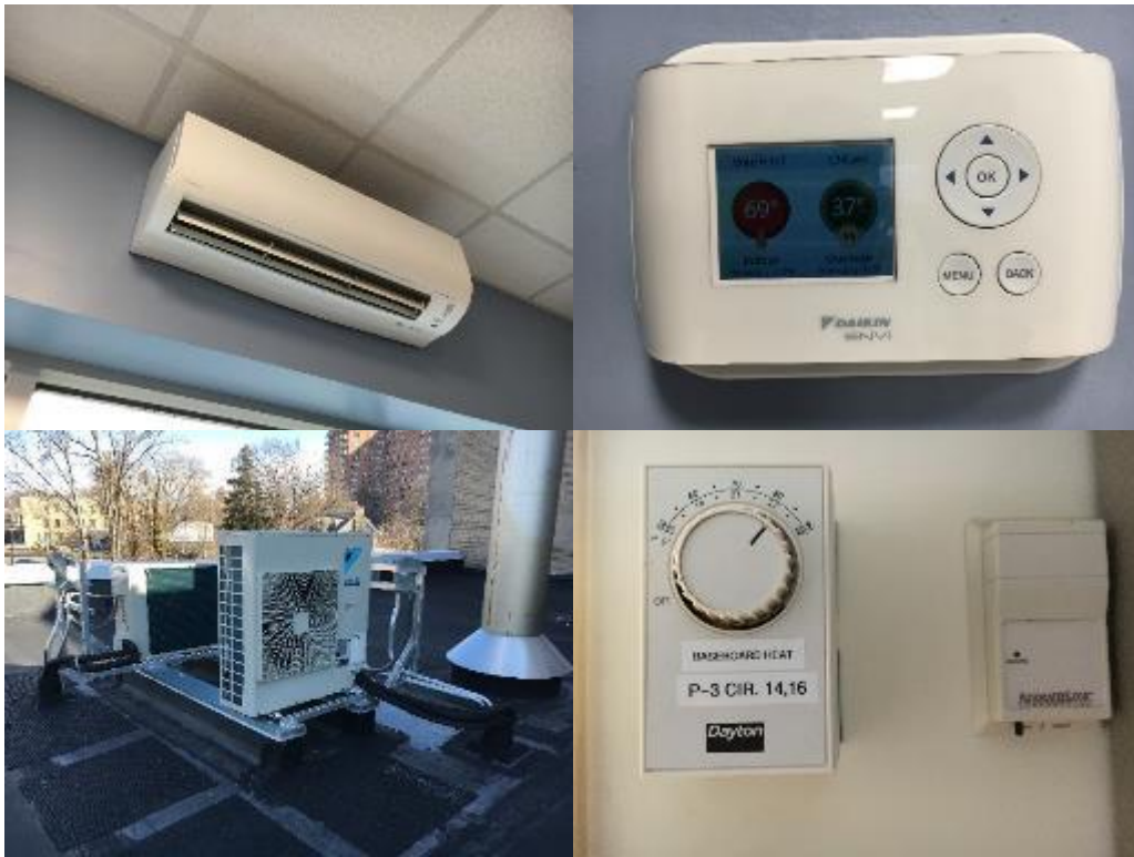
Image 22: Split Heat Pump Systems and Controls
