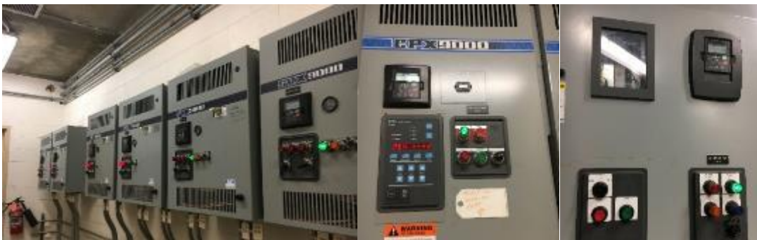
Image 10: Variable Frequency Drives
