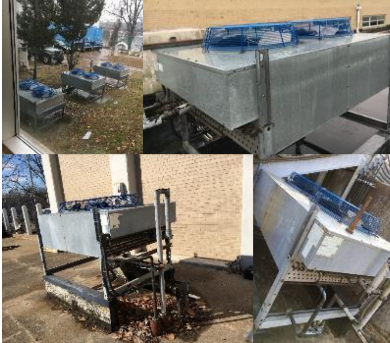
Image 20: Remote Condensing Units for RTUs
