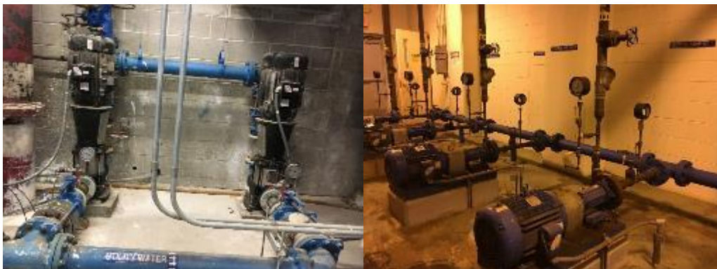
Image 7: Raw Water and High Service Pump Motors
