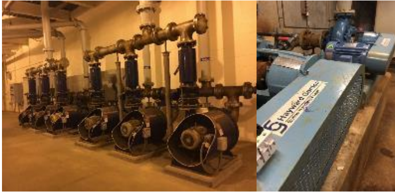
Image 9: Vacuum Pump and Solid Handling Pump Motors
