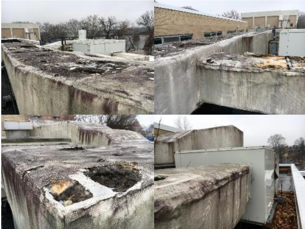
Image 15: Ductwork Insulation in Poor Condition
