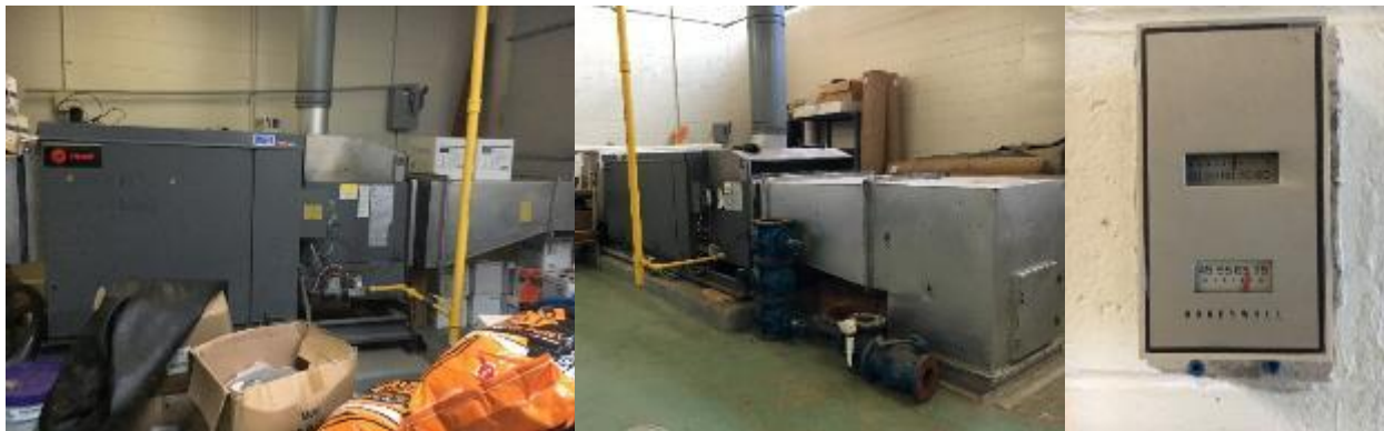
Image 16: Gas Fired Forced Air Furnaces with Remote Condensing Units in MDF
