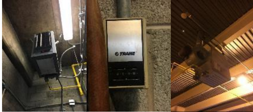
Image 17: Gas Unit Heaters and Local Manual Controls
