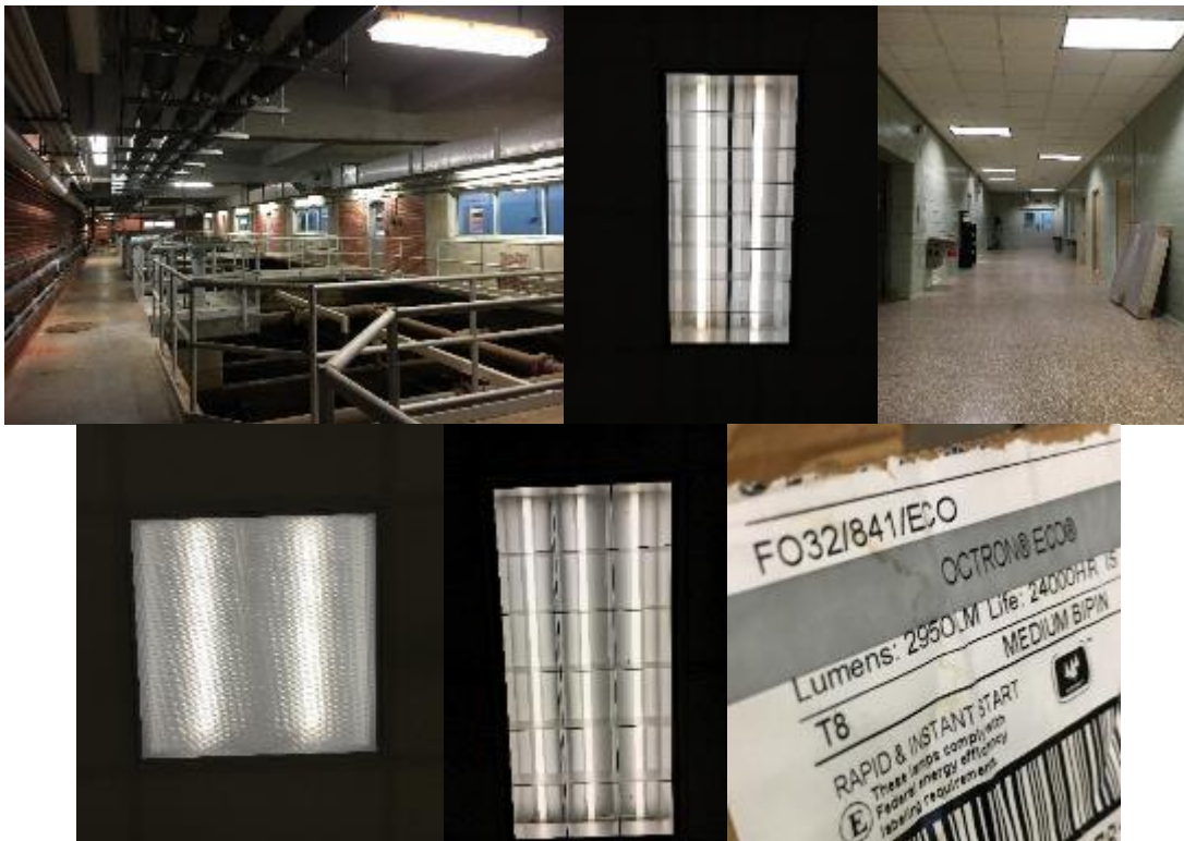
Image 1: Interior Linear Fluorescent T8 Light Fixtures
