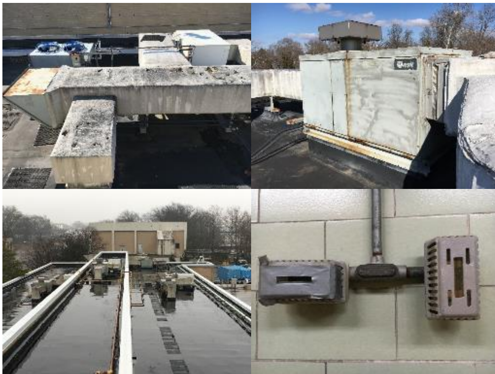
Image 14: Gas Fired Forced Air Furnaces with Remote Condensing Units on Roof of Filtration Plant
