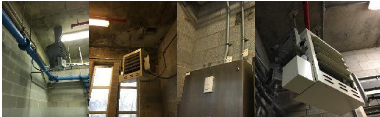
Image 18: Electric Unit Heaters and Local Manual Controls
