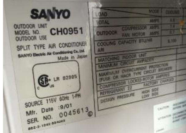
Image 9 – DX split system nameplate
