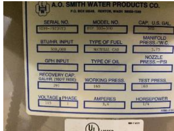
Image 11 – Water heater nameplate
