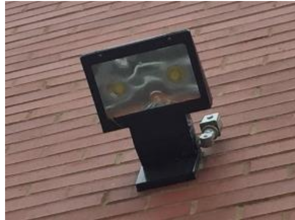
Image 3 – Exterior LED fixture
