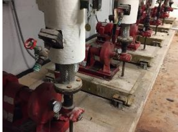
Image 5 – Hot Water Pumps
