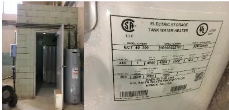
Image 10: Domestic Water Heating
