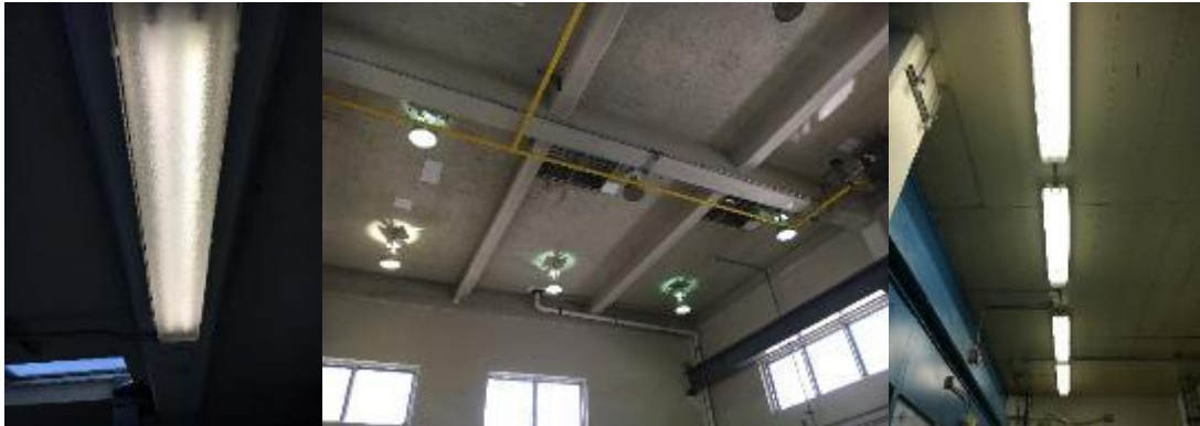
Image 2: Interior Lighting Systems
