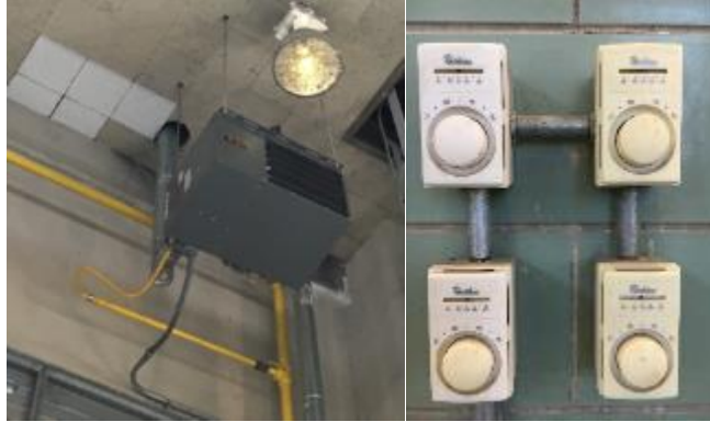
Image 4: Gas Unit Heaters and Manual Dial Thermostats
