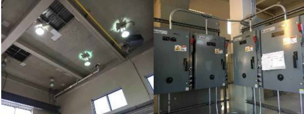
Image 6: Dampers and Exhaust Fan Switches
