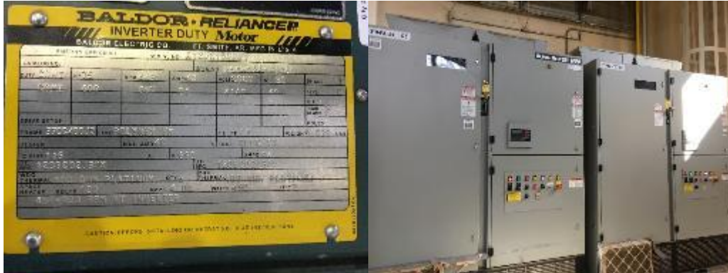
Image 8: Process Pump Two Speed Motor Nameplate and Drives
