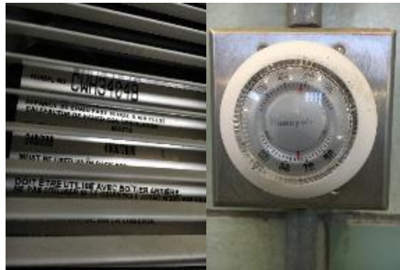
Image 5: Electric Unit Heater and Manual Dial Thermostat in Office
