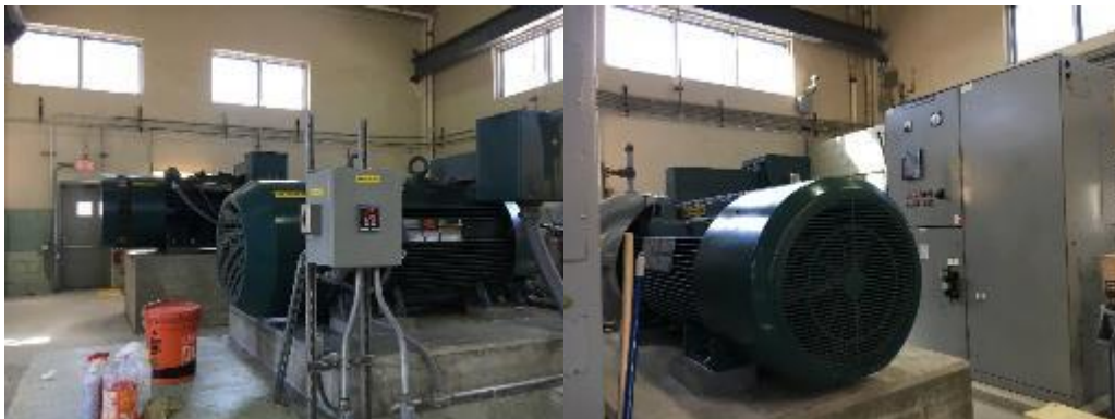
Image 7: Process Pump Two Speed Motors
