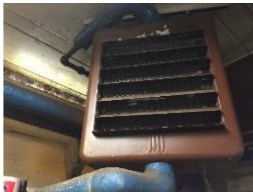
Image 7: Hot Water Unit Heater
