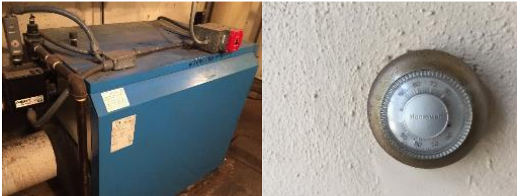
Image 6: Hot Water Heating System in Main Sewage Pumping Station
