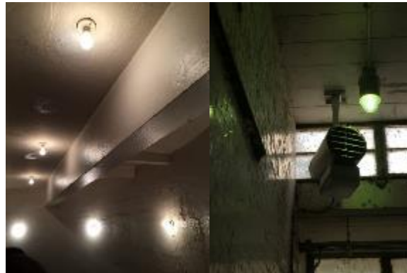
Image 3: Interior Lighting Systems
