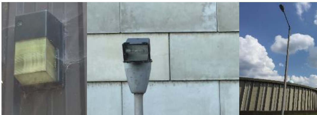
Image 4: Exterior Lighting Systems
