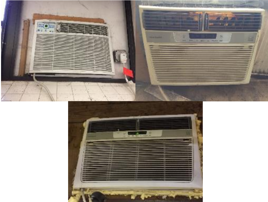
Image 12: Electric through Wall AC Units
