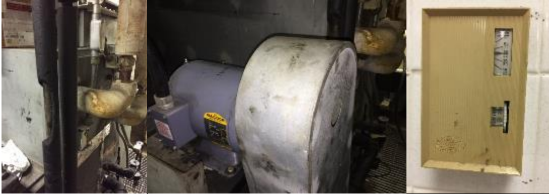
Image 8: Air Handling Unit with Manual Thermostat Control
