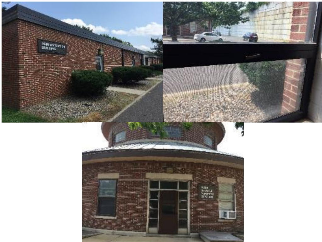
Image 1: Building Envelope (Administration Building and Main Pump House)
