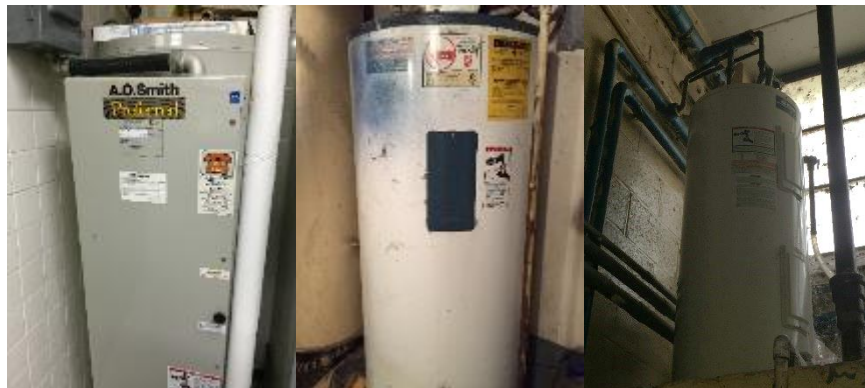
Image 13: Domestic Hot Water Systems
