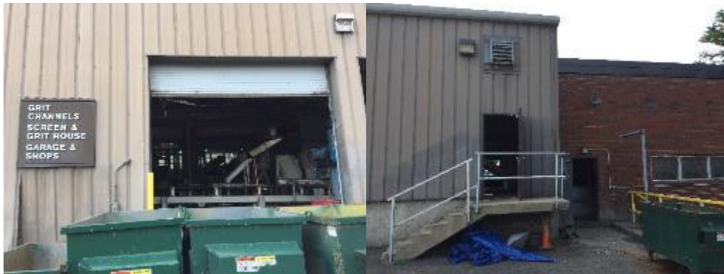
Image 2: Building Envelope (Screening Grit Station)
