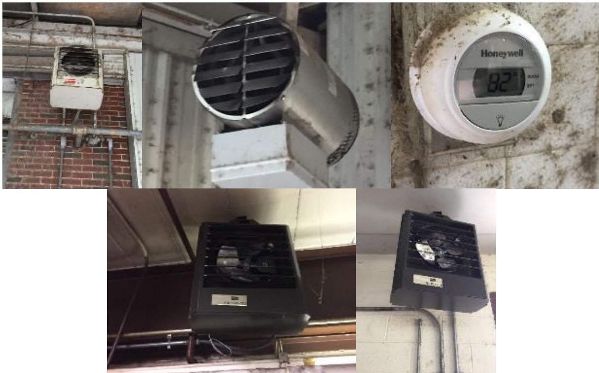
Image 11: Electric Unit Heaters and Local Manual Controls
