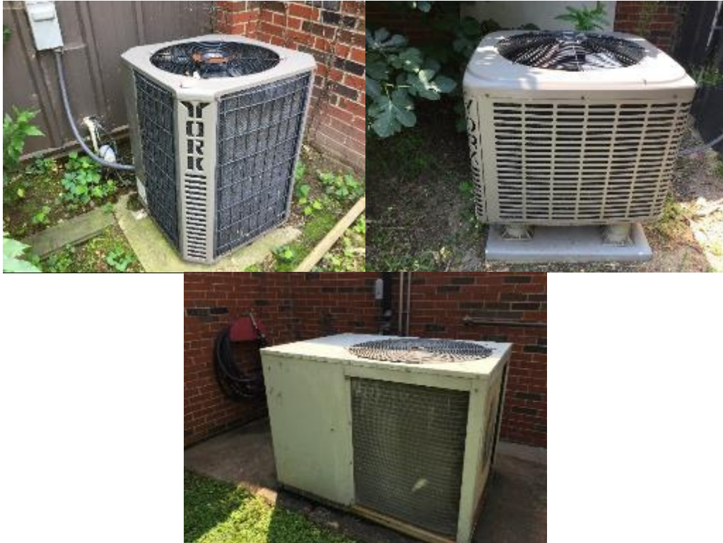
Image 10: Remote Condensing Units at Administration Building
