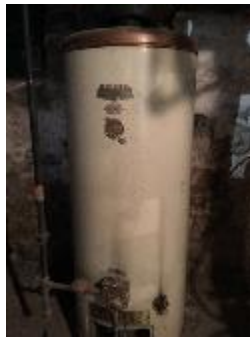
Figure 11 – Domestic Hot Water Equipment
