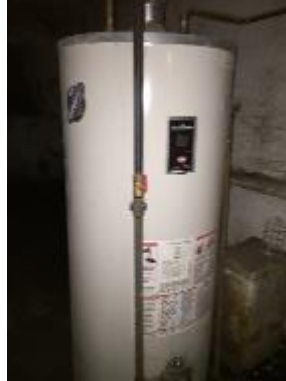
Figure 11 – Domestic Hot Water Equipment
