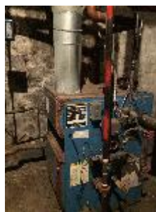
Figure 9 – Heating Hot Water Equipment
