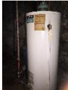
Figure 10 – Domestic Hot Water Equipment
