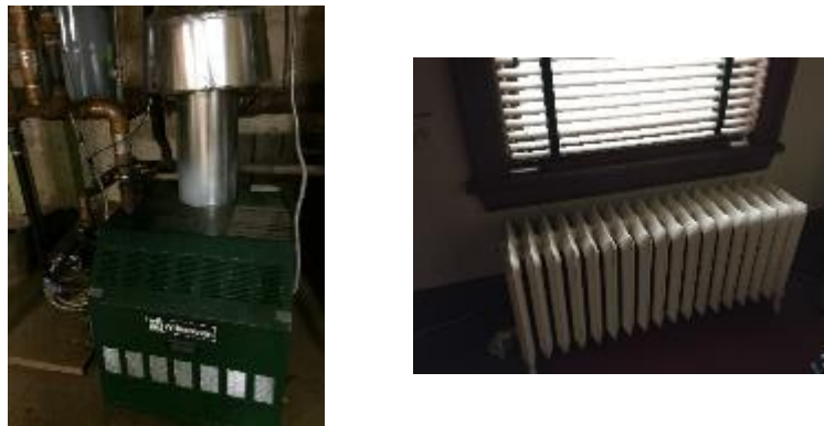
Figure 9 – Heating Hot Water Equipment
