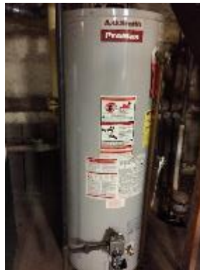
Figure 11 – Domestic Hot Water Equipment
