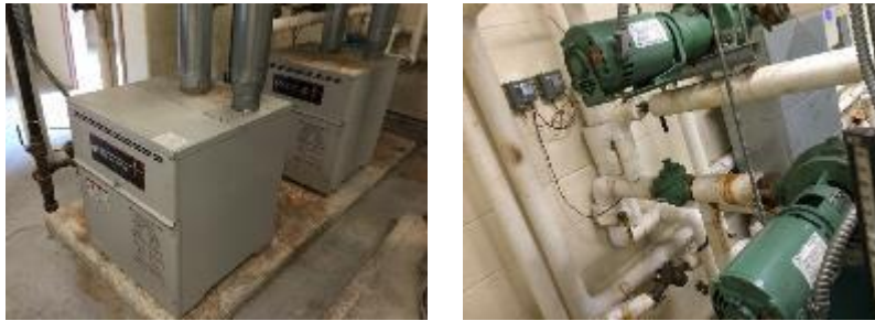
Figure 9 – Heating Hot Water Equipment
