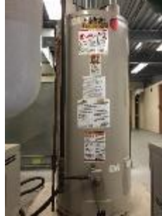
Figure 11 – Domestic Hot Water Equipment
