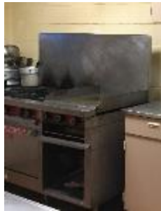
Figure 12 – Food Service Equipment
