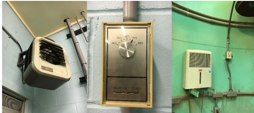
Image 7: Electric Unit Heaters and Thermostats
