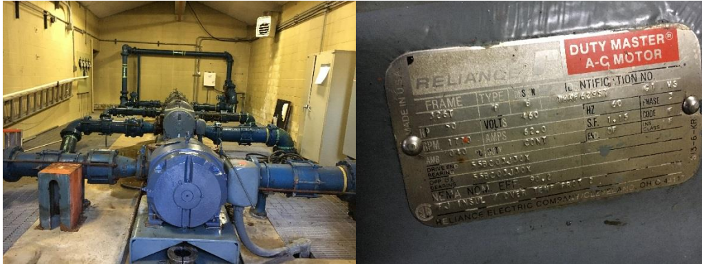
Image 4: Scotch Road (Ewing Township) Water Pumps and Motors
