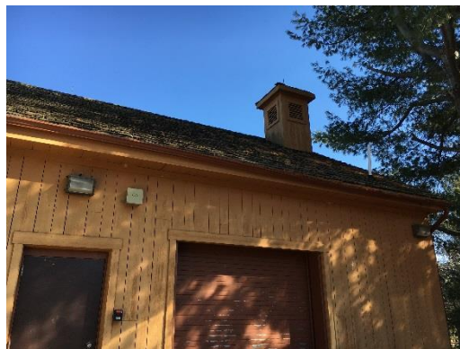
Image 3: Exterior Lighting Fixtures
