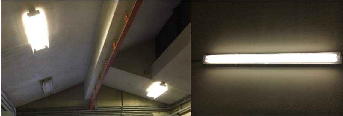
Image 2: Interior Lighting Fixtures
