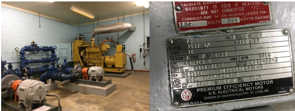
Image 5: Denow Road (Hopewell Township) Water Pumps and Motors
