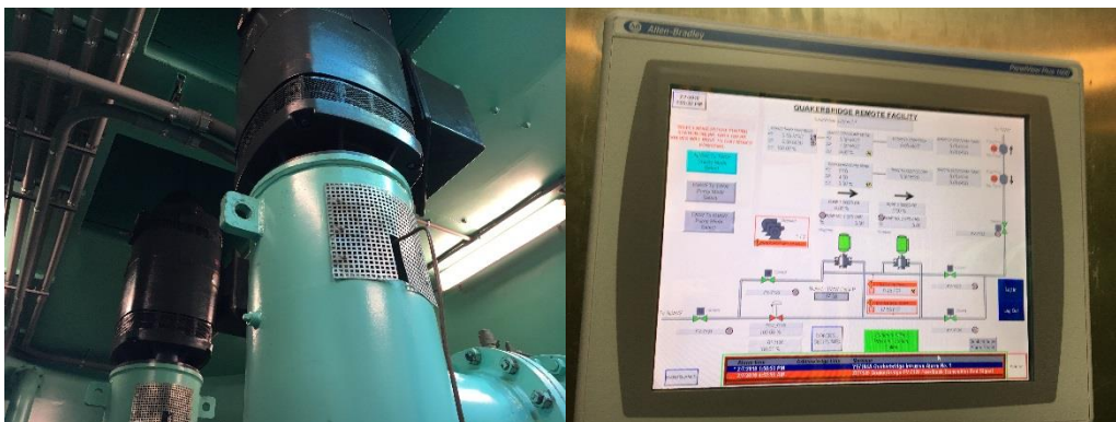
Image 6: Quakerbridge Road (Lawrence Township) Water Pumps and Motors
