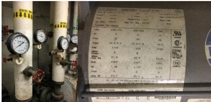
Heating hot water pump motors
