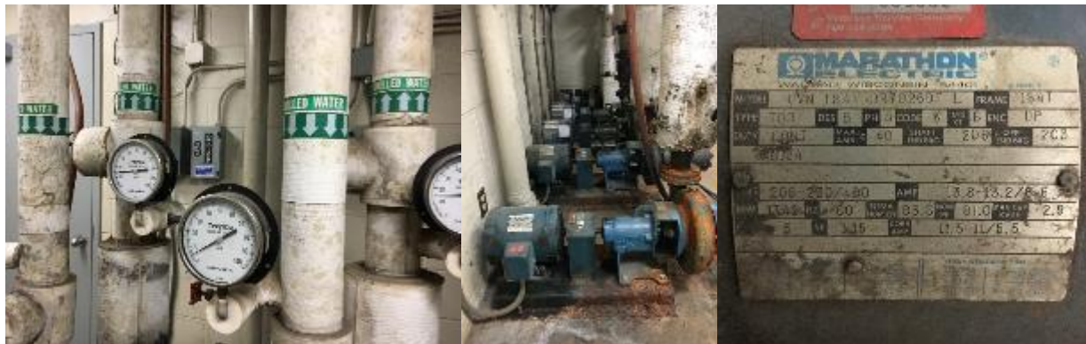
Chilled water pump motors
