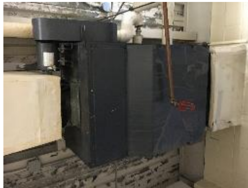
Air Handling Unit for Locker Room
