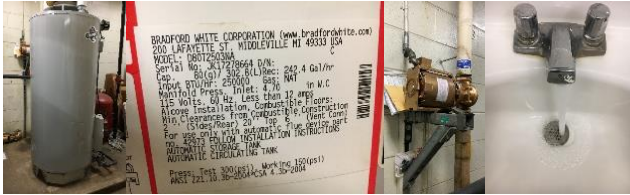
DHW Heater, Circulation Motor and High Flow Faucet Aerator
