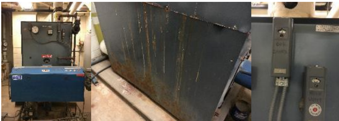
Hot Water Boiler
