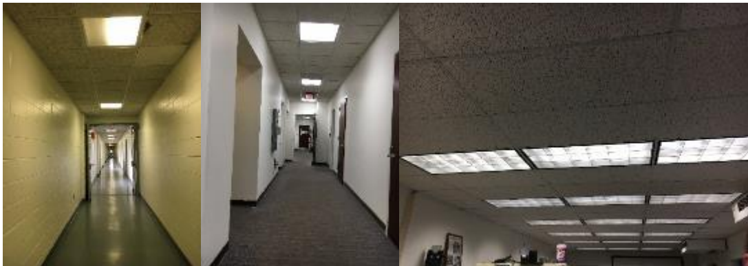
Comparison in light quality, T8 vs LED in Hallways
