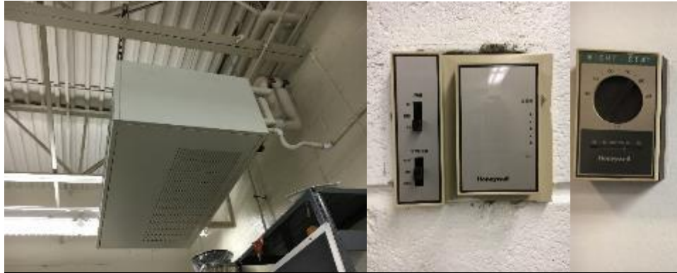
Ceiling PTAC and Basic Manual Dial Thermostat Control
