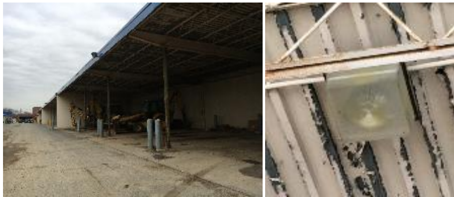
Exterior HID lighting in Garage Bays (Wall Mounted Floods and Surface Mounted Canopy)
