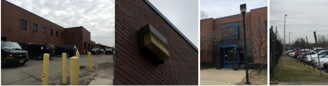
Exterior HID lighting (Building Mounted and Pole Mounted)
