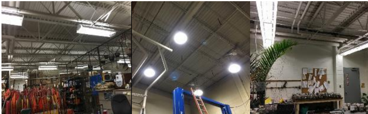
Warehouse T8 lighting and Mechanic's Shop HID lighting
