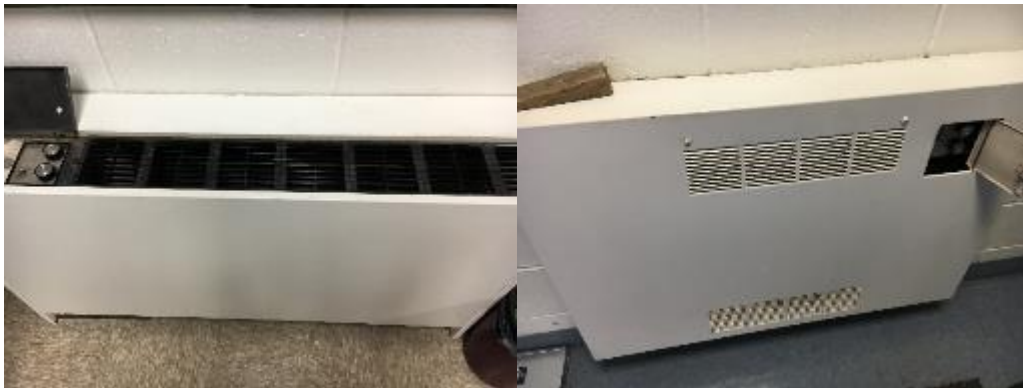
Terminal PTAC and Cabinet Unit Heater
