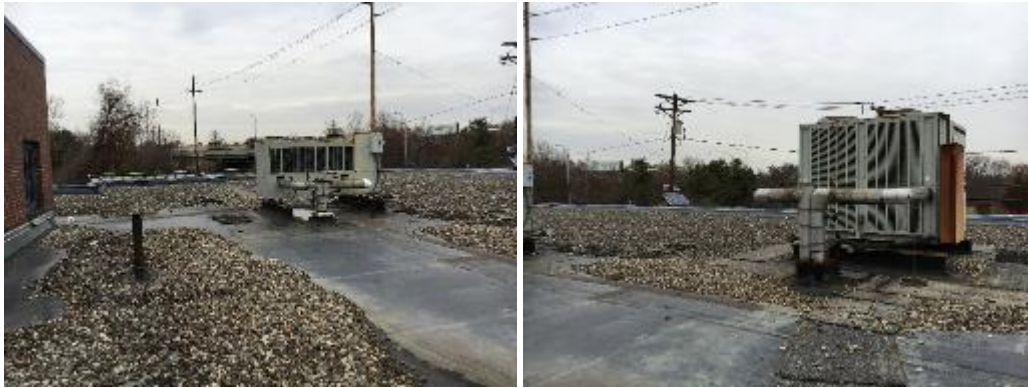
Air Cooled Scroll Chillers
