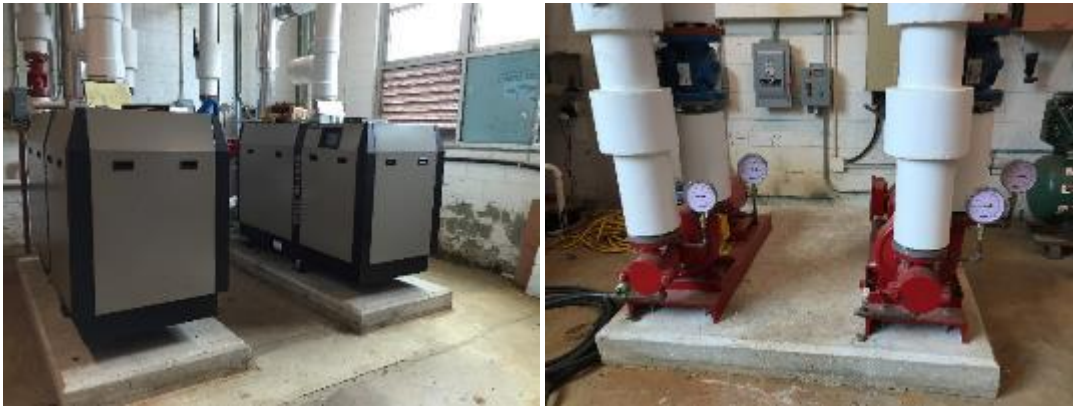
Image 3 Hot water system
