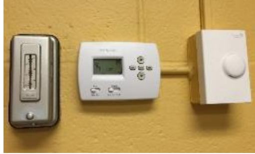
Image 4 Air conditioning system
