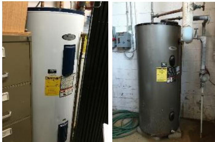
Image 5 Domestic hot water heater
