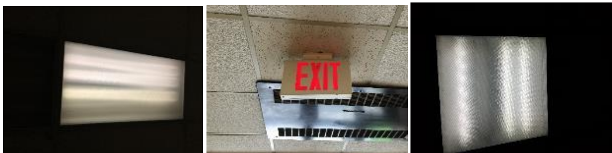
Image 2 Typical lighting fixtures
