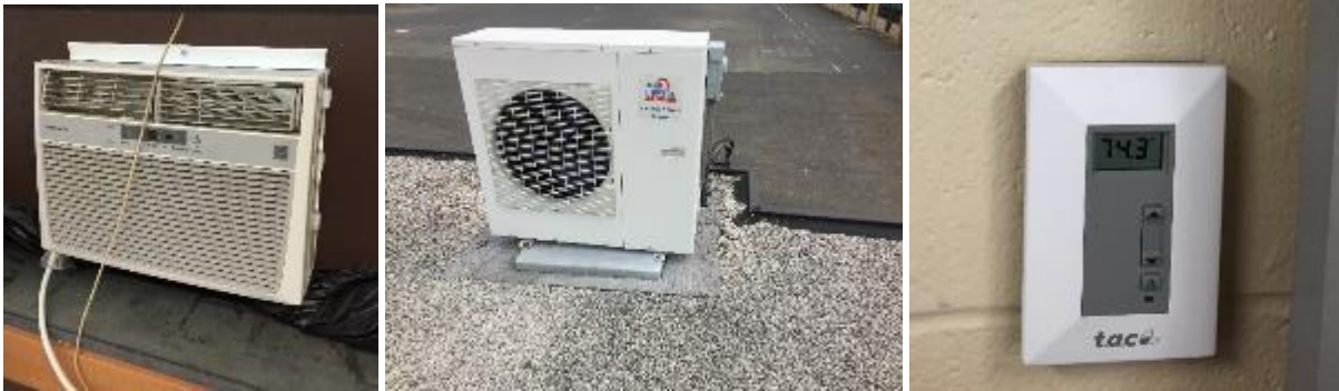
Image 4 Air Conditioning System
