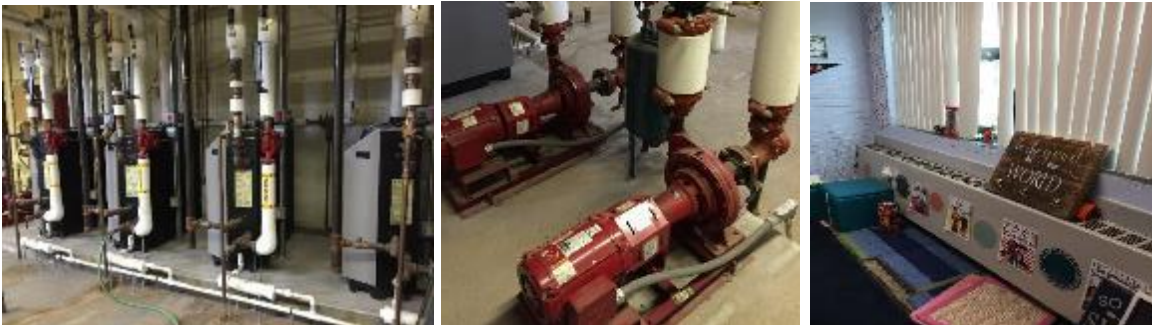
Image 3 Hot Water System
